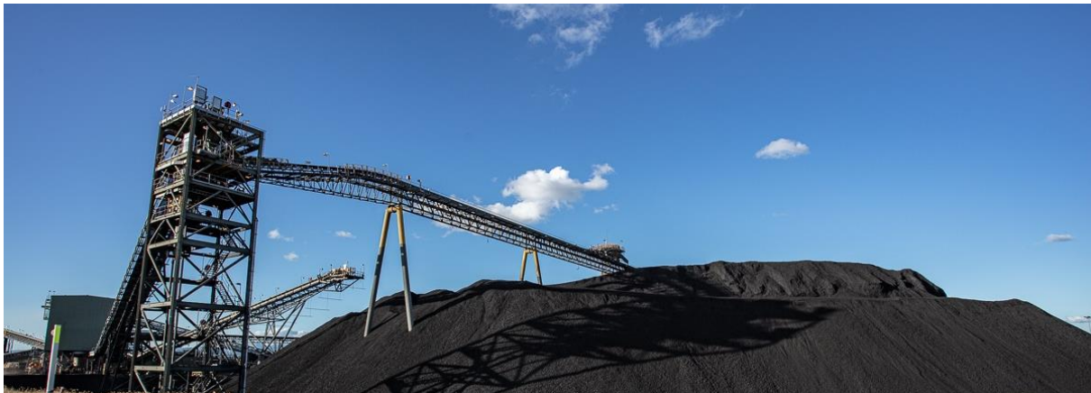
Plate 2-3 Existing Product Coal Stockpile
