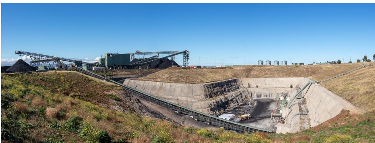
Plate 2-1 Narrabri Mine Box Cut and Drifts
