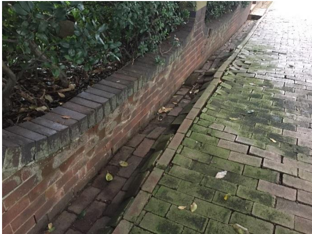
Figure 17. The brick box drain along the Avenue facing northwest
