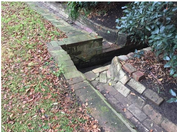
Figure 21. The edging of the brick guttering runs into drainage
