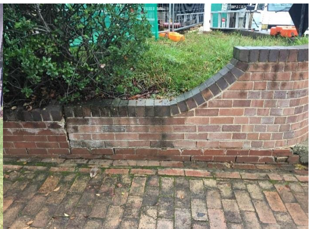
Figure 28. Soil putting pressure on the retaining wall that borders the former offices, facing south west
