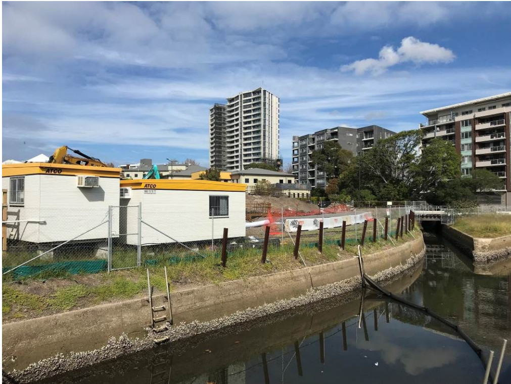
Photo Plate 3: Looking south-east towards site with Cottage Creek in foreground
