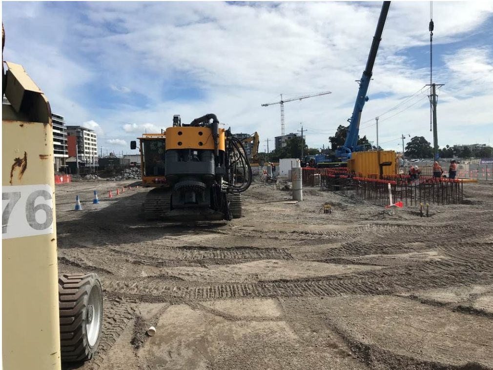
Photo Plate 1: Looking west towards construction site
