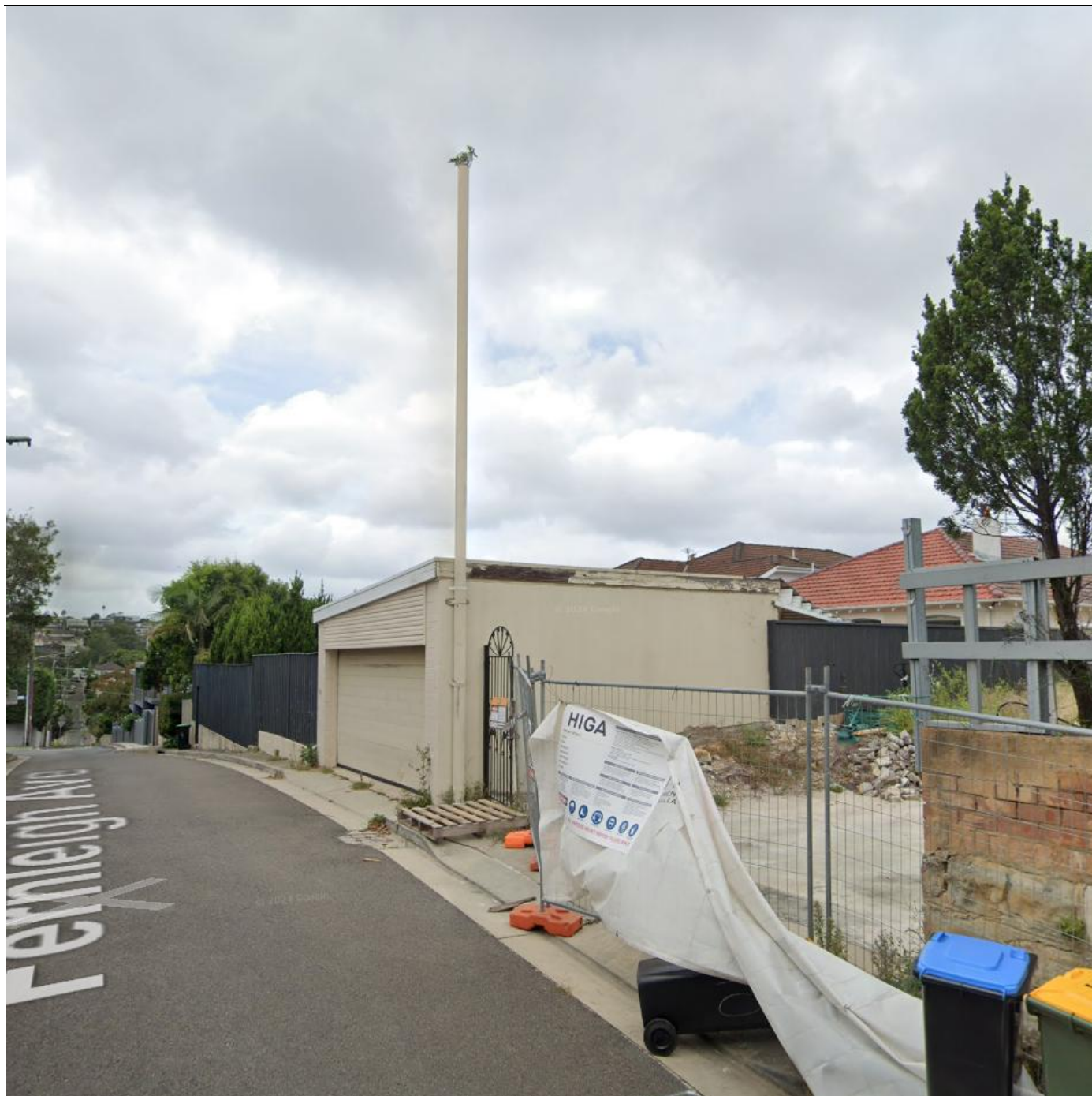
Figure 8: Sewer Vent Shaft (Source: Google Maps)
