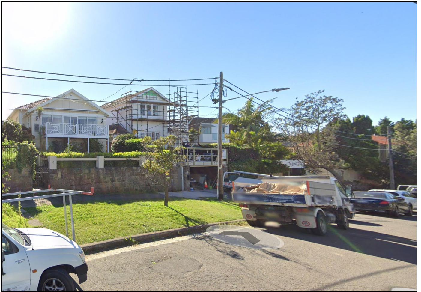
Figure 3:Overhead Ausgrid and Optus Infrastructure in Vicinity of the New Development (Source: Google Maps)
