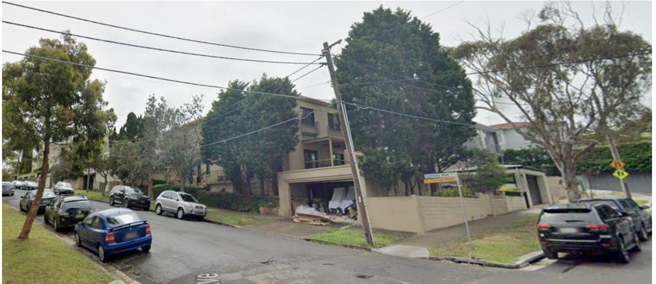
Photo of site; 2A/ 2-6 CONWAY AVENUE & 38-40 CARLISLE STREET, ROSE BAY
