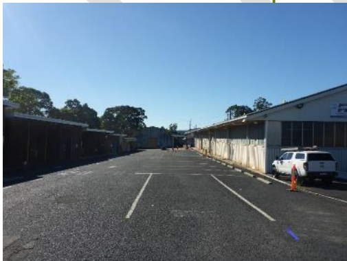
Figure 8: View north showing several of the warehouses and bitumen card park
