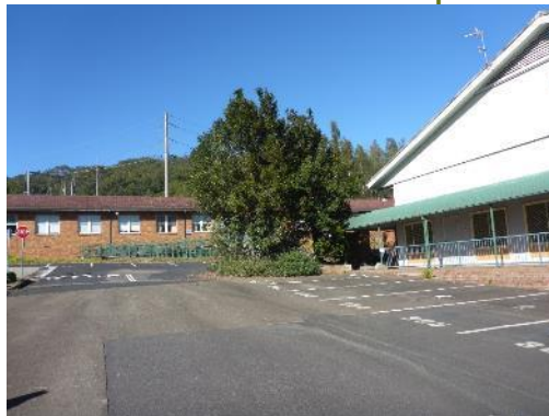
Figure 9: View south east of several of the warehouses and bitumen card park
