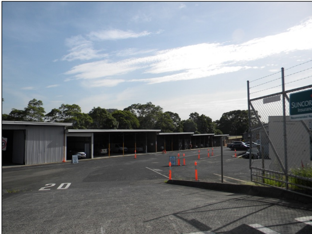
Figure 4: The site as viewed from the entrance off Faunce Street West.
