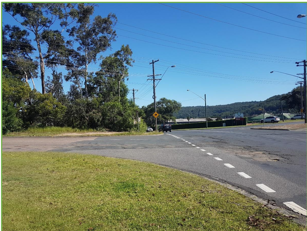
Intersection of Racecourse Road and Faunce Street West (east)
