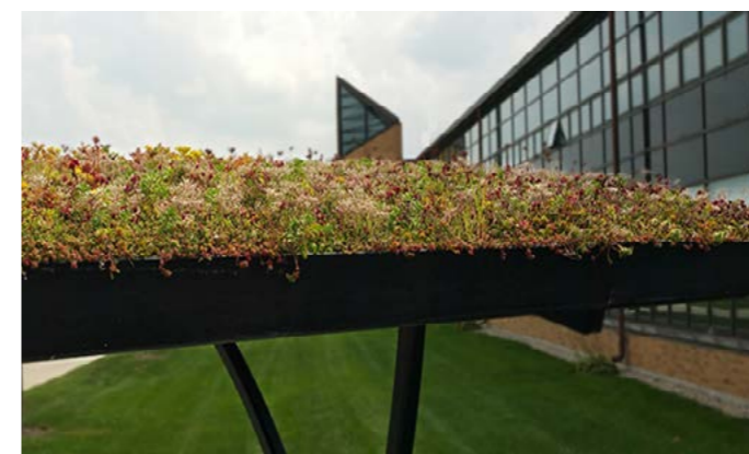
Shelters - Cantilevered steel structure with green roof
