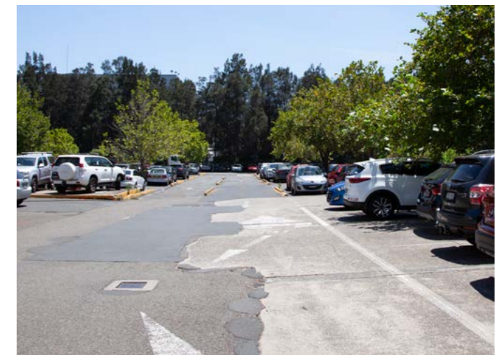
Asphalt and concrete surfacing
