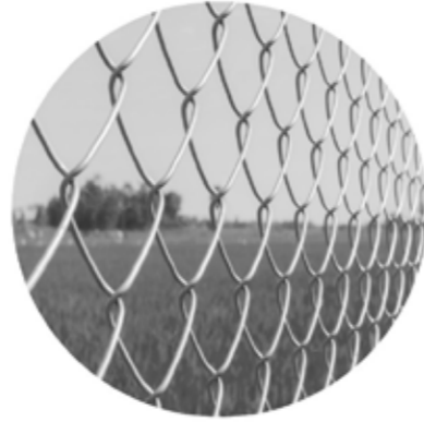
Carpark : Chainwire Mesh Facade Colour; Galvanised finish
