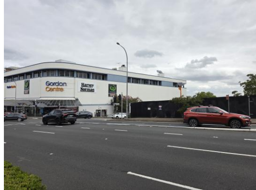
Pacific Highway looking south-west (site is on the right)
