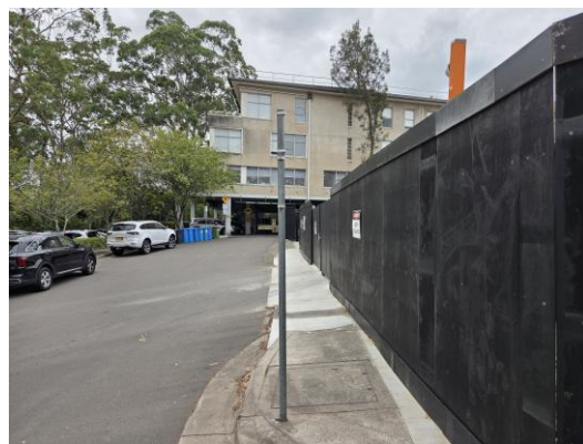
Radford Place looking north towards Ku-ring-gai Council Chambers (site is on the right)
