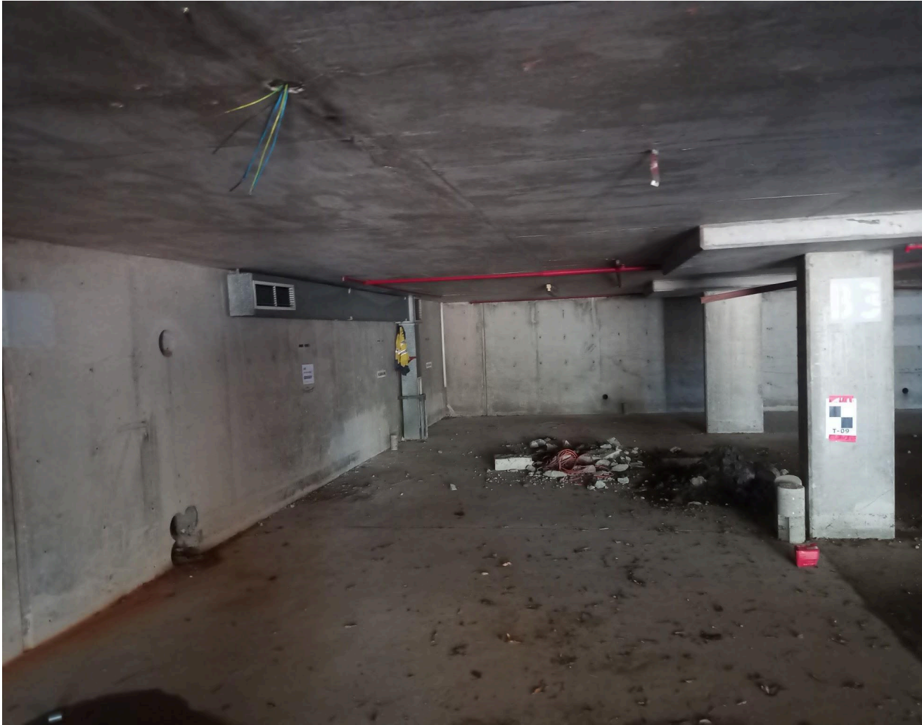
Photo 4 - representative image of the internal structure of the semi-demolished structure
