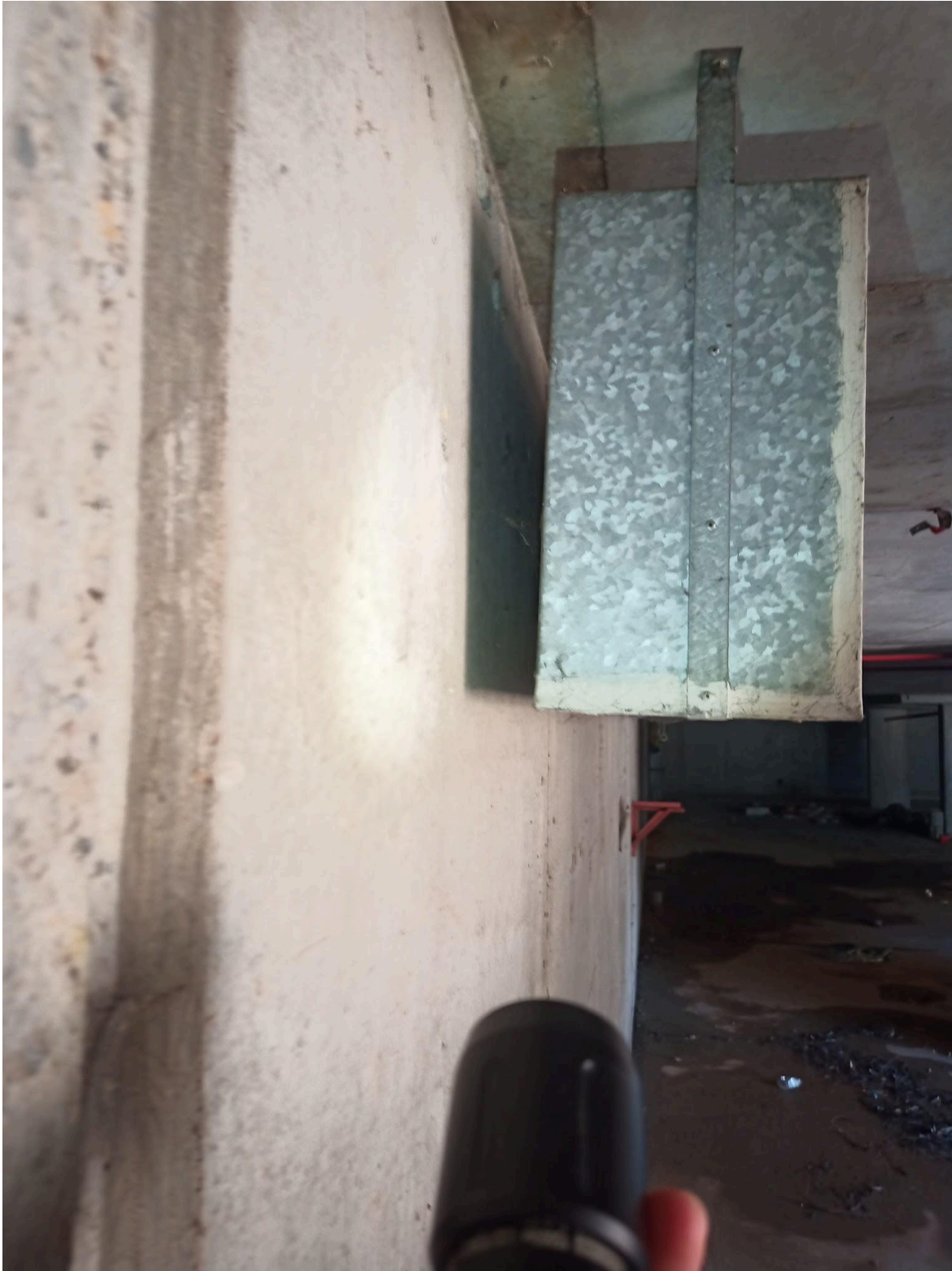
Photo 6 - Inspection of possible bat roosting locations behind derelict air vets undertaken throughout the semi-demolished structure
