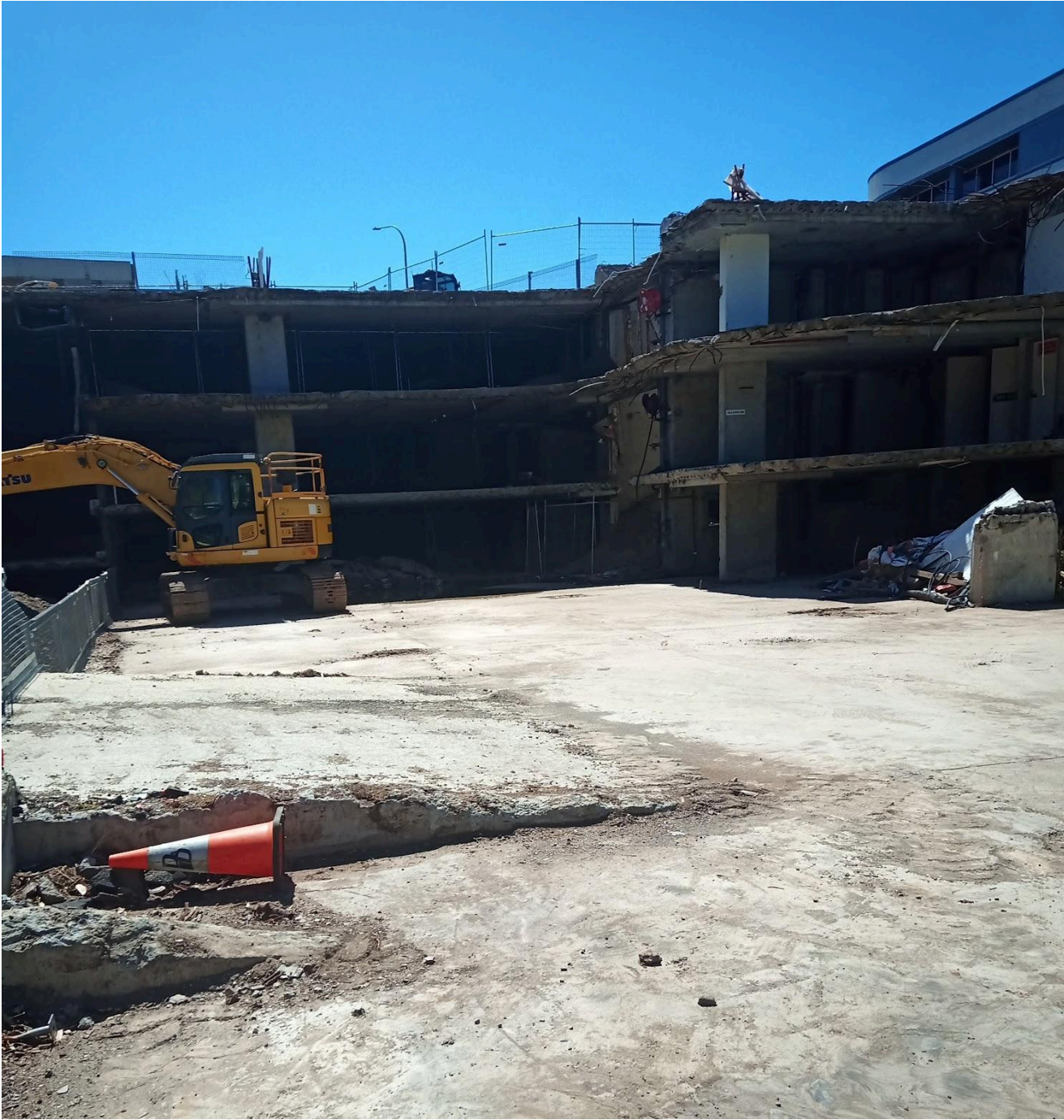
Photo 3 - Semi-demolished car park facility in the centre of the site
