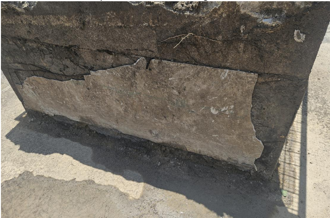
Compressed Concrete Sheeting- Not ACM
