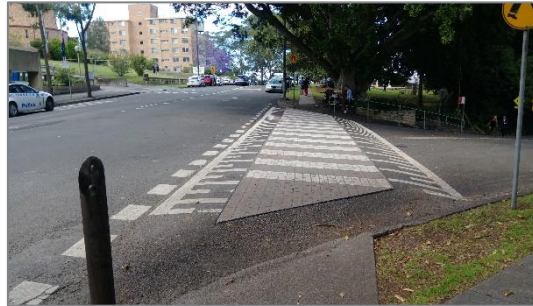
Figure 3.6: Vaughan Avenue (facing south)
