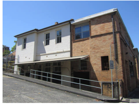
Plate 25: The building today. (JCHD 0420)
