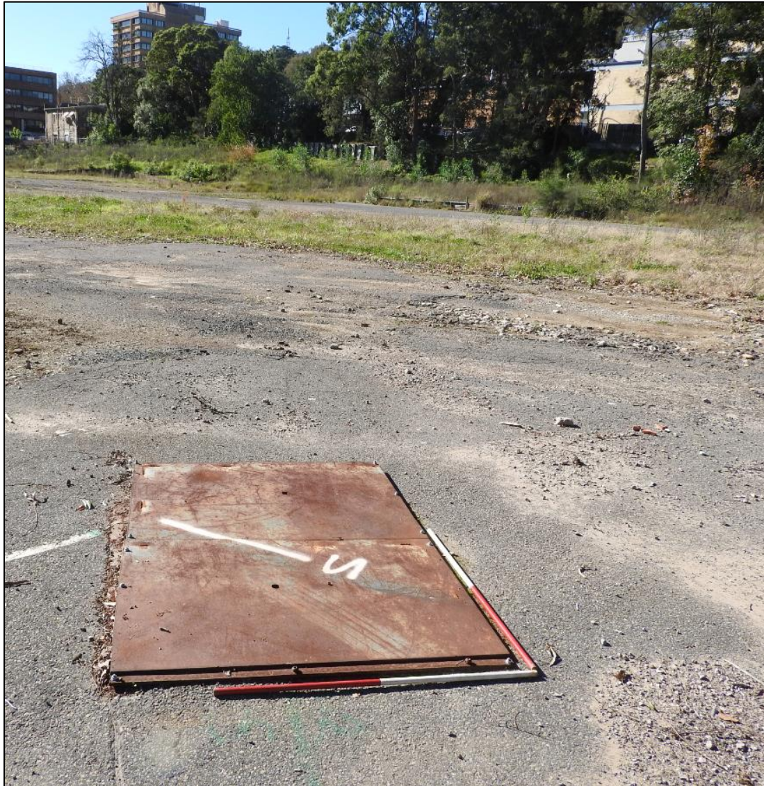
Figure 5.6 Manhole for services, facing north east. Note photograph taken prior to any excavation works. AMAC Group - DSCN0430 (06/02/2017)
