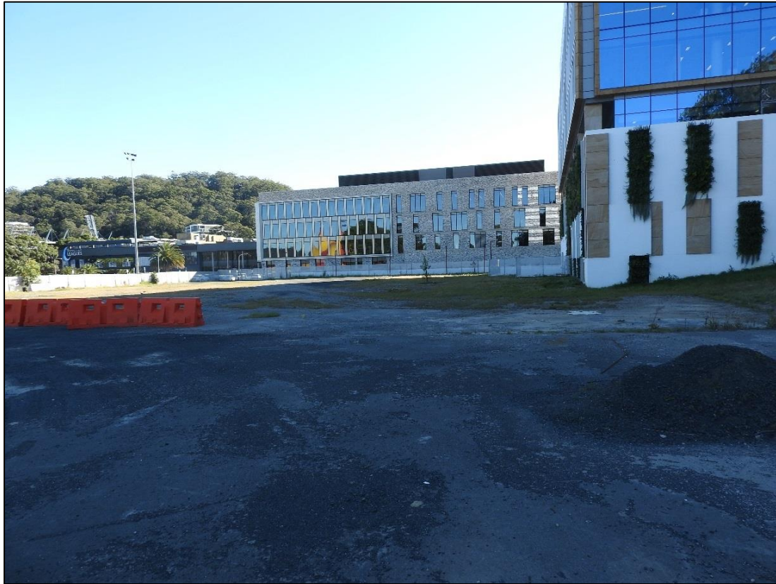
Figure 5.2 Northern end of study site (Unit 2). Facing north. AMAC, 22 nd August 2019, digital image DSCN3114.
