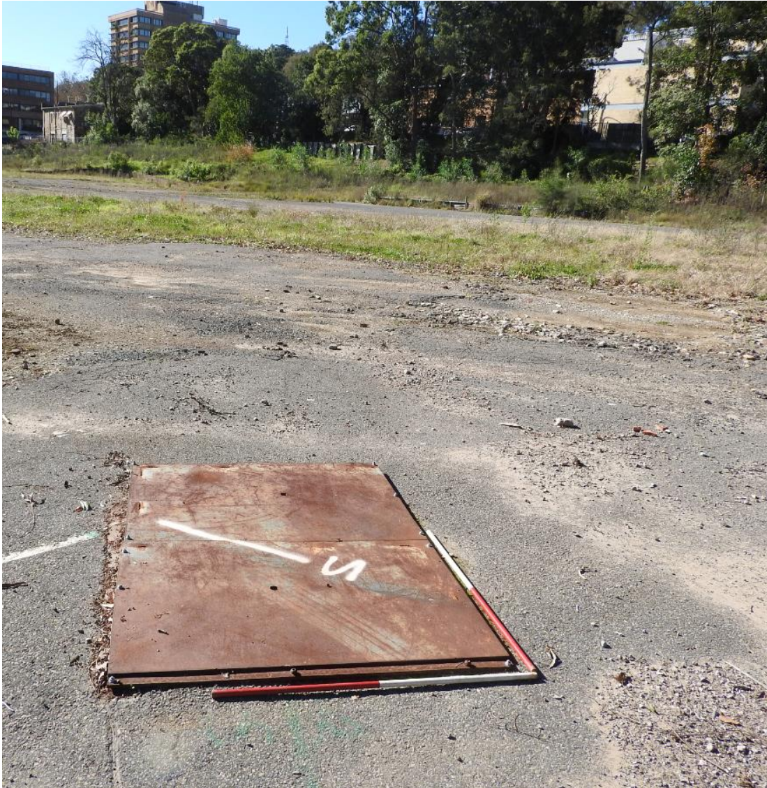
Figure 3.6 Manhole for services, facing north east. Note photograph taken prior to any excavation works. AMAC Group - DSCN0430 (06/02/2017)
