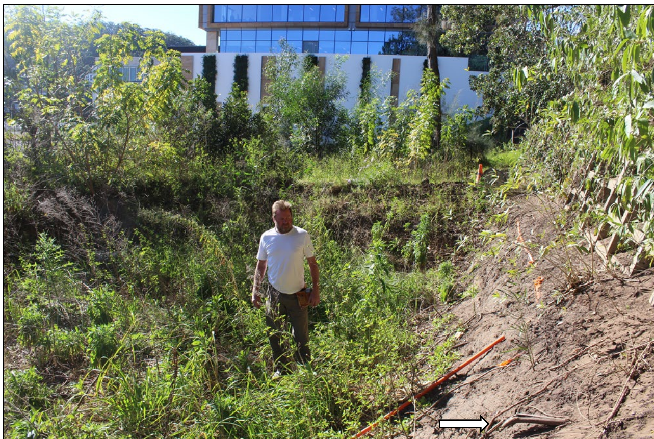
Plate 1 —Illustrates the location of an existing excavation approximately 8m x 4m x 1.5m, and approximately 5m west of the subject fig. Note severed/torn roots at right (arrowed)
