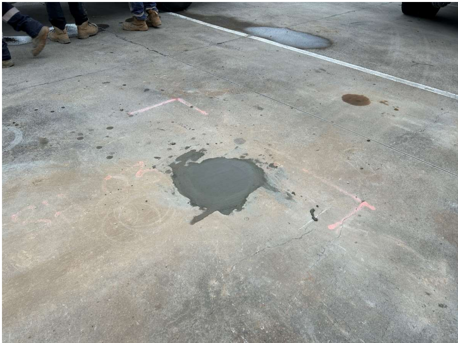
Photo 12 - Typical backfilled borehole (BH03)
