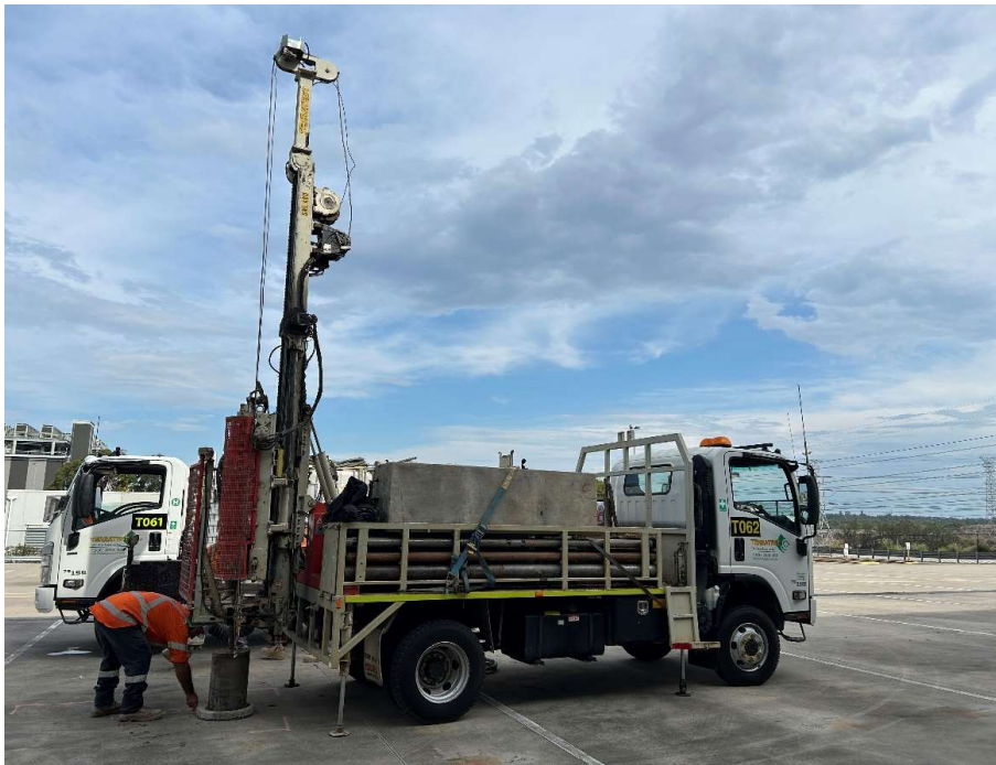
Photo 6 - Machine used for drilling (MCT200)
