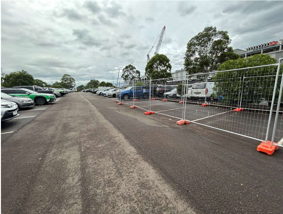
Photo 13 - General site photo looking north from BH-G
