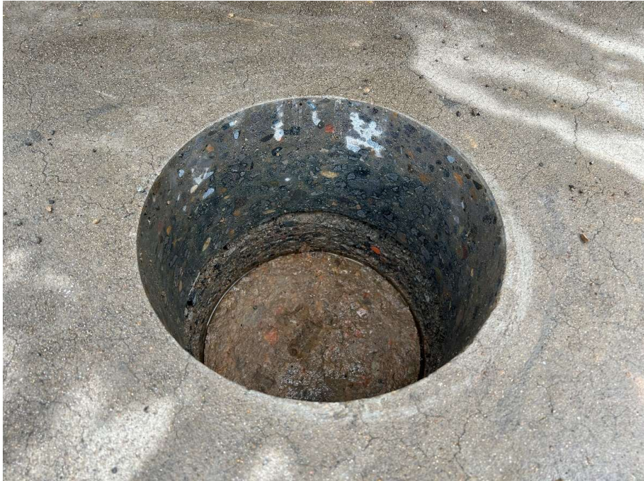
Photo 11 - Typical borehole after concrete coring (BH03)
