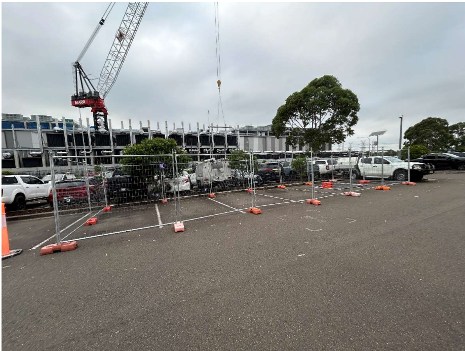
Photo 14 - General site photo looking east from BH-H
