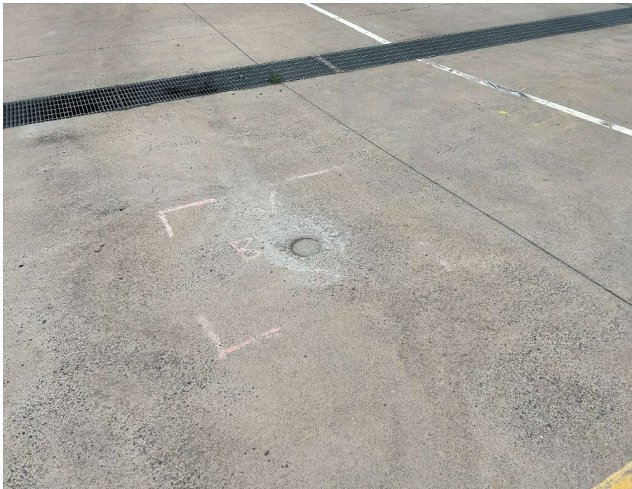
Photo 16 - Typical backfilled borehole (BH-B)
