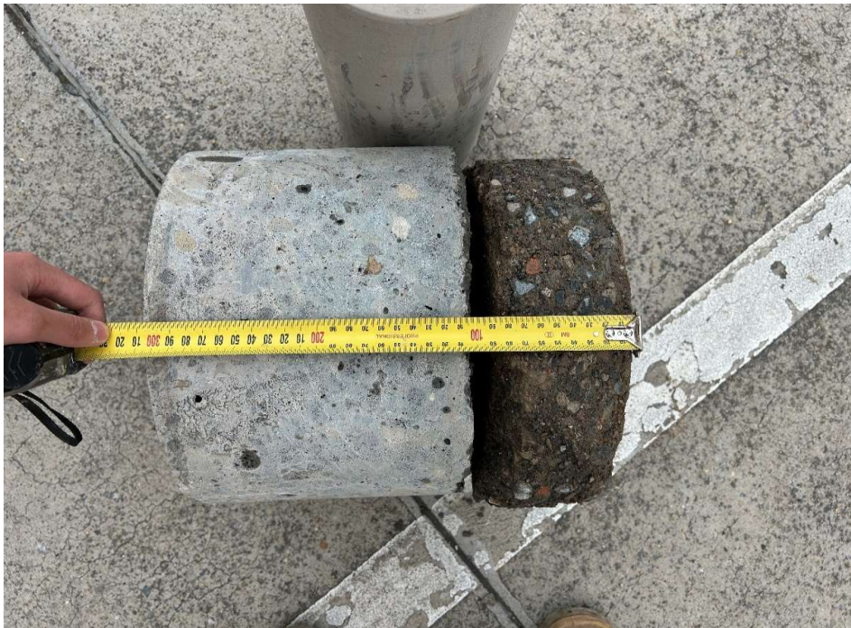
Photo 10 - Typical core of concrete pavement (BH03)
