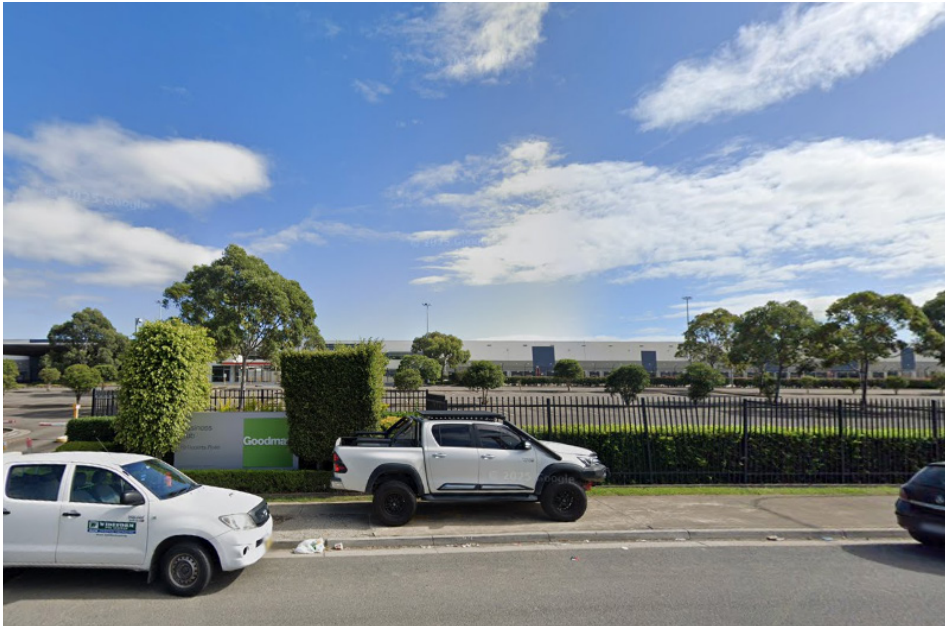
02 STREET VIEW LOOKING TOWARDS NORTH WEST FROM ROBERTS ROAD
