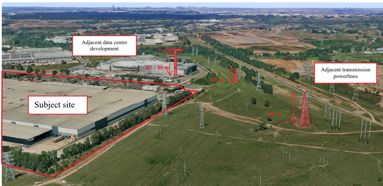
Figure 9: height estimation of crane works at site relative to adjacent structures and reference points
