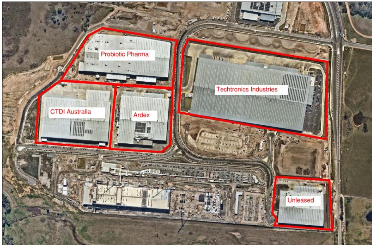
Figure 3: Nearby developments (Source: Nearmap)
