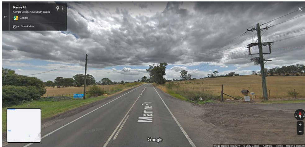
Low voltage and 11 kV high voltage overhead power lines (including pole mounted substation no. 8418 to the opposite side of Mamre Road. The extended low voltage overhead service conductor goes to a customer owned / private pole on 757-769 Mamre Road (Lot 22 DP 258414) providing the customer connection for the existing buildings on that lot.
