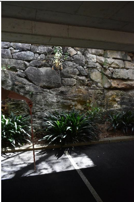
Figure 19: Sandstone retaining wall – sandstone block additions
