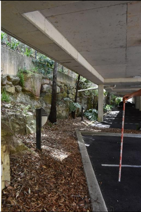
Figure 19: Sandstone retaining wall – sandstone block additions
