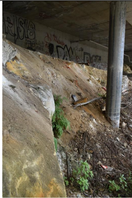
Figure 30: Foundations at eastern end of the office building, and ceramic drainage pipes
