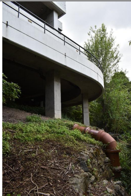
Figure 30: Foundations at eastern end of the office building, and ceramic drainage pipes
