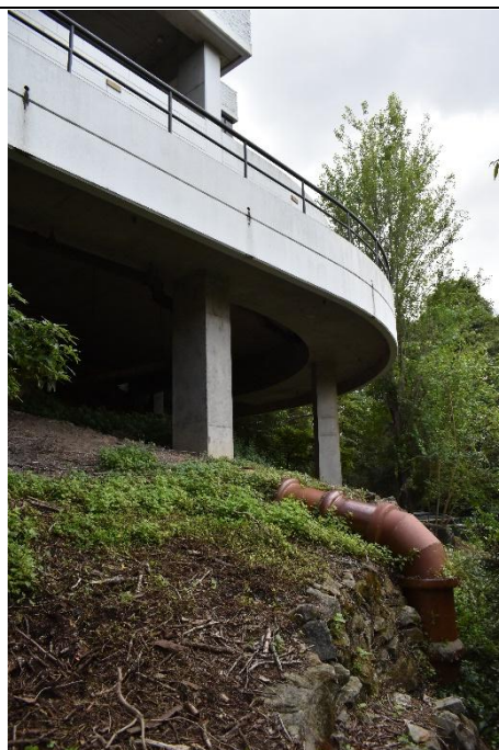
Figure 14: Foundations at eastern end of the office building, and ceramic drainage pipes
