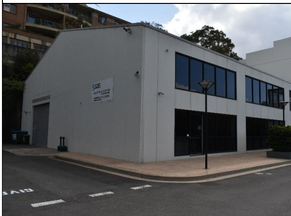
Figure 11: North view of warehouse
