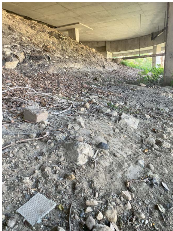
Photograph 8: Area beneath suspended slab under eastern end of car park area, facing north east, FCS fragment in foreground (9 September 2024).
