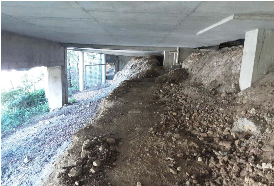
Photograph 4: Photo of area beneath suspended slab, facing west (9 September 2024).
