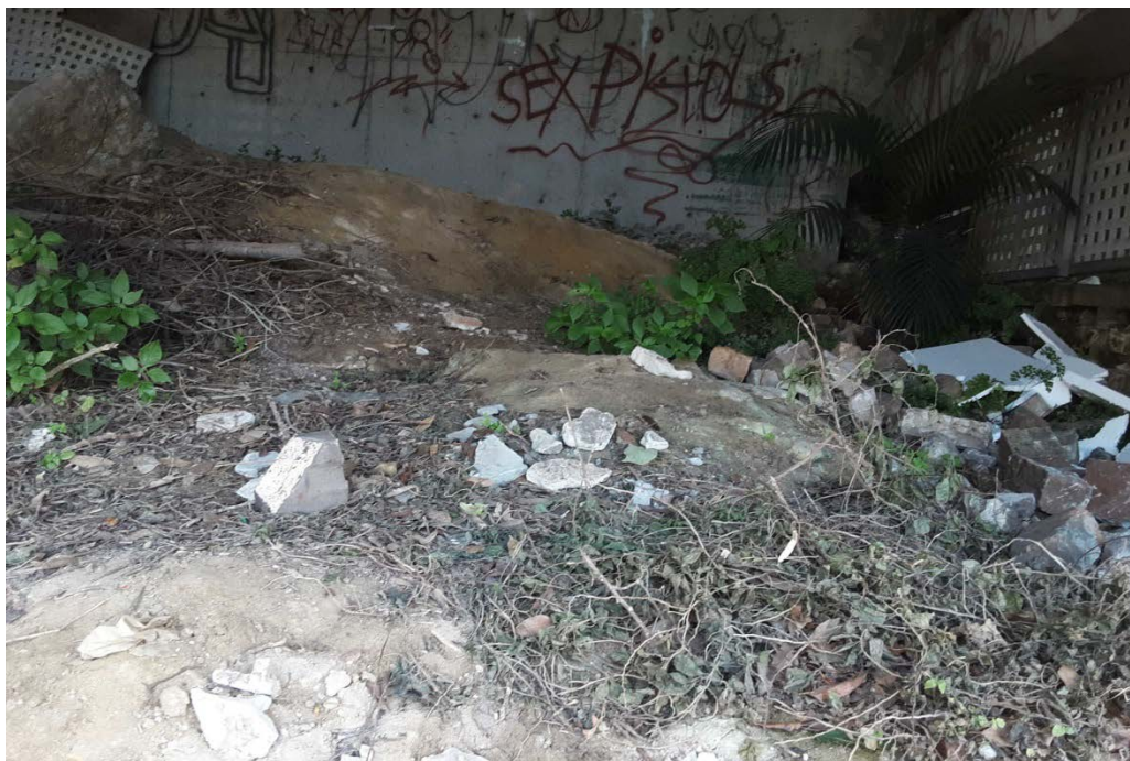
Photograph 6: Photo of area beneath suspended slab under eastern end of car park area, facing north. (9 September 2024).
