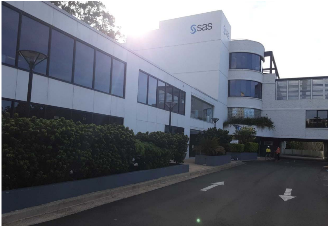
Photograph 1: Site overview, building frontage, facing north-east (9 September 2024)
