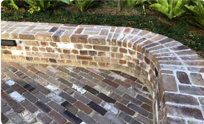
Recycled brick seating wall
