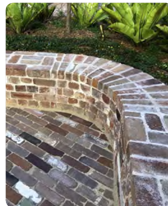
Recycled brick seating wall
