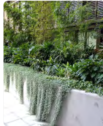
Concrete planter walls
