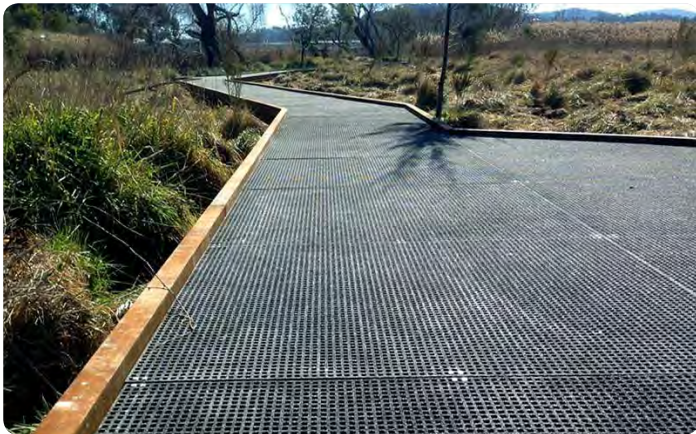
Raised FRP decking over Ephemeral zone
