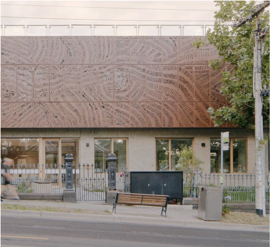
Melbourne Indigenous Transition School Boarding House by McIlldowie Partners
