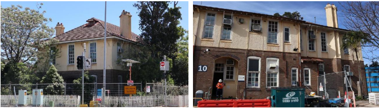
Figure 14 Photos of Mowbray House (Source: Tropman and Tropman)
