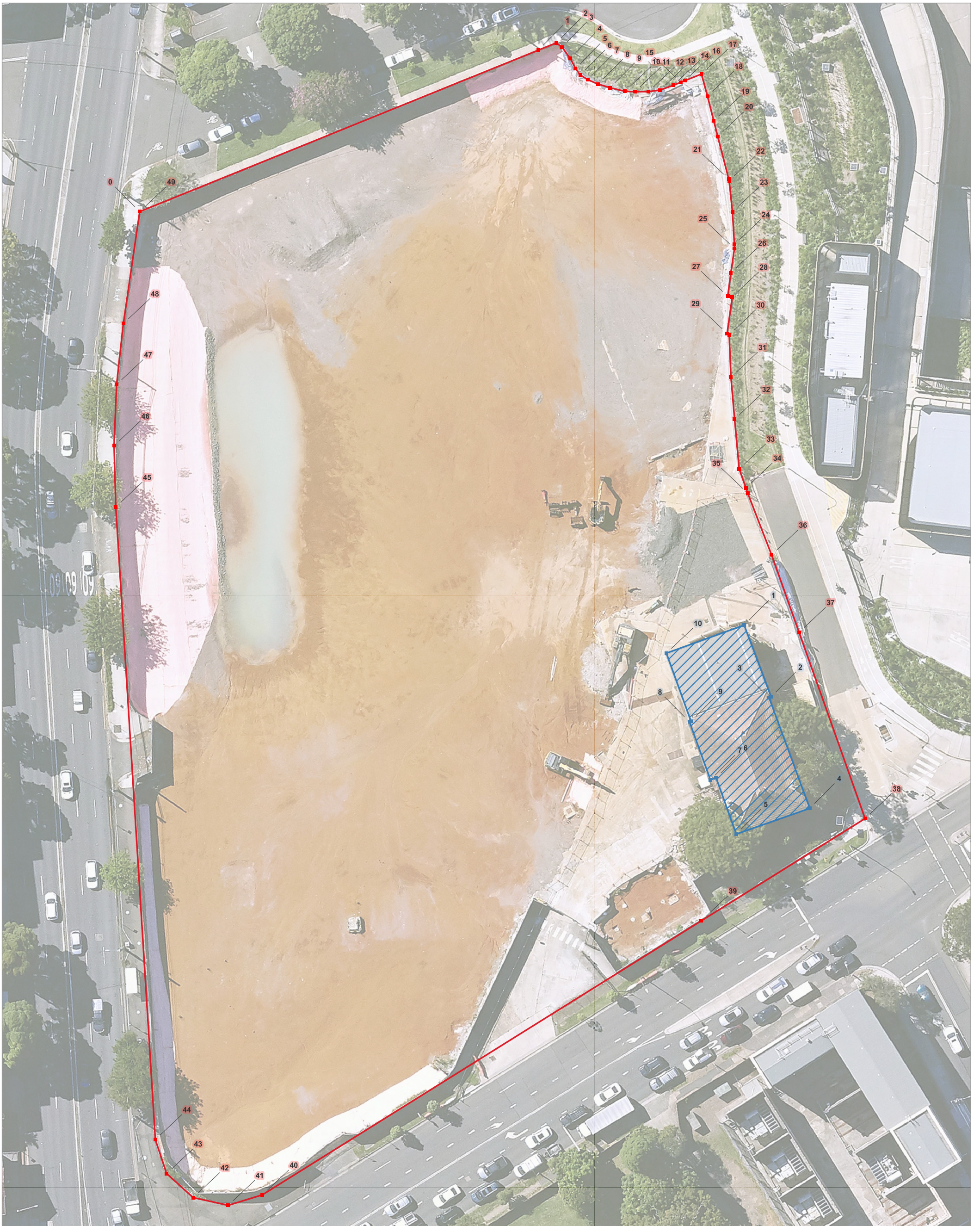
Figure 10: Final Site Audit Boundary Chatswood Metro Dive Site Validation Report
