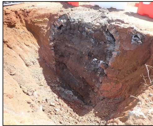
Figure 4.6 Beehive cistern, post excavation.
