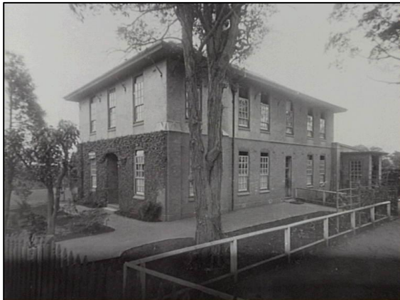
Figure 3.16 Main entry to the Mowbray House School building, n.d. (Source: Picture Willoughby, File No: 6536/6536552).
