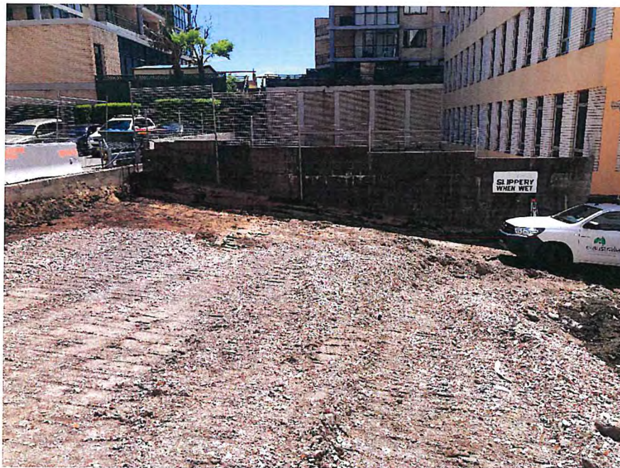
Photo 2: General site condition, looking southwest (09/01/2019)
