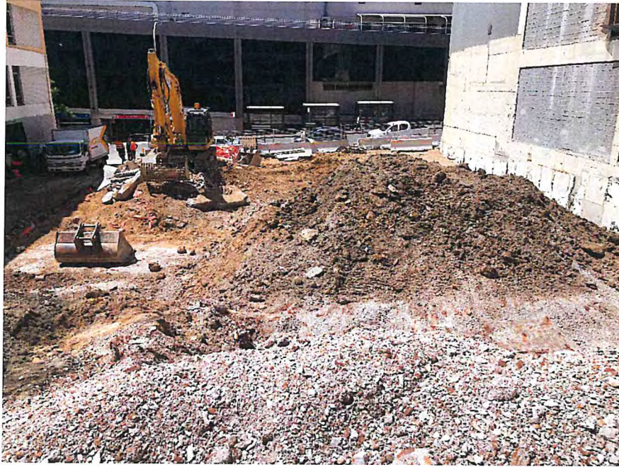
Photo 3: General site condition, looking southwest (09/01/2019)
