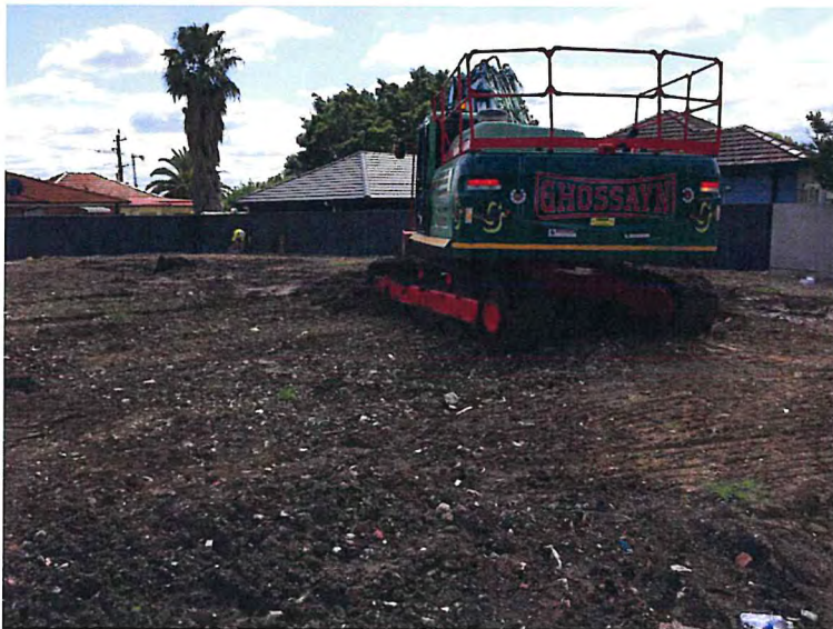
Photo 2: View of site conditions, looking east.
