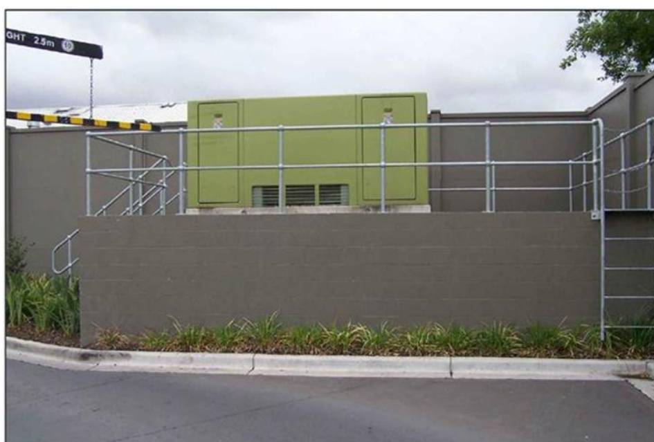
Figure 51 - Example substation raised above 1:100 flood level
