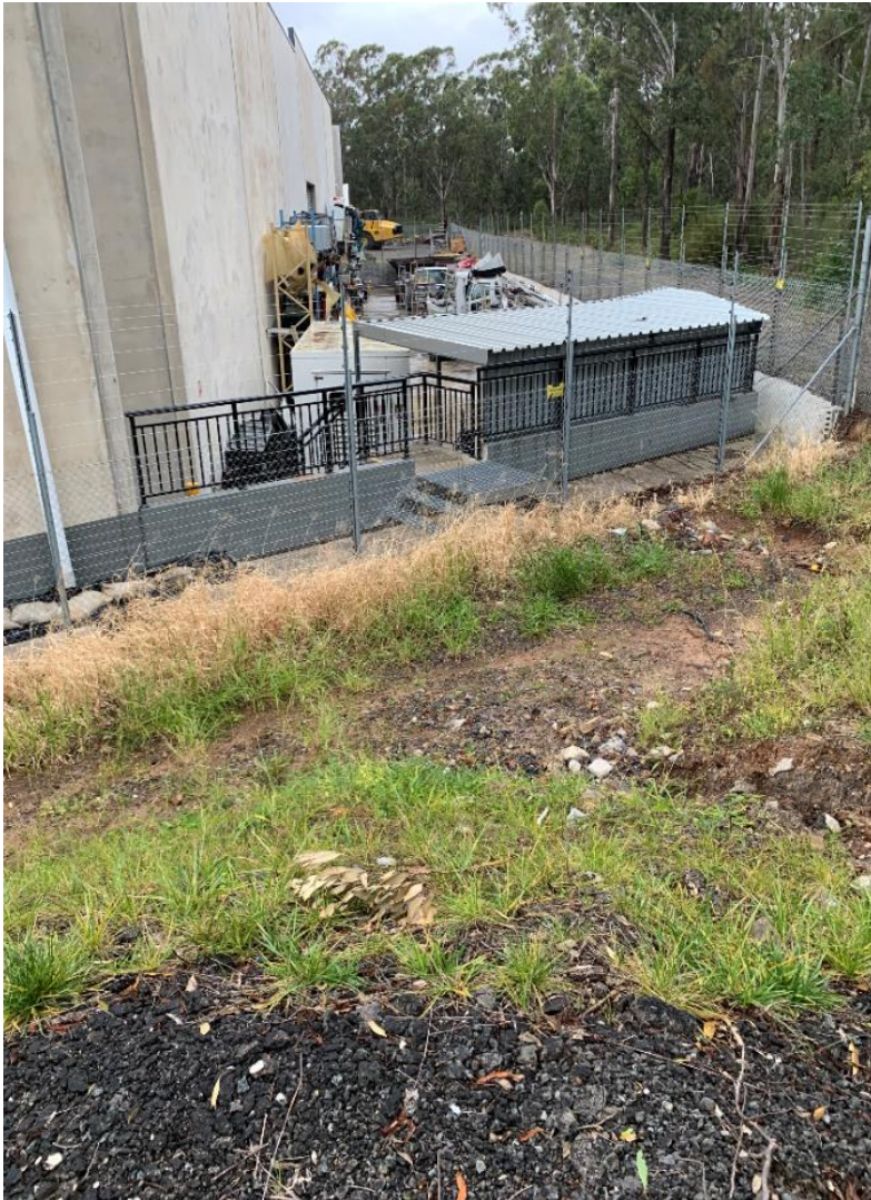
Figure 6 Photo of Swale Drain at Boundary with No.10 Raceway Place
