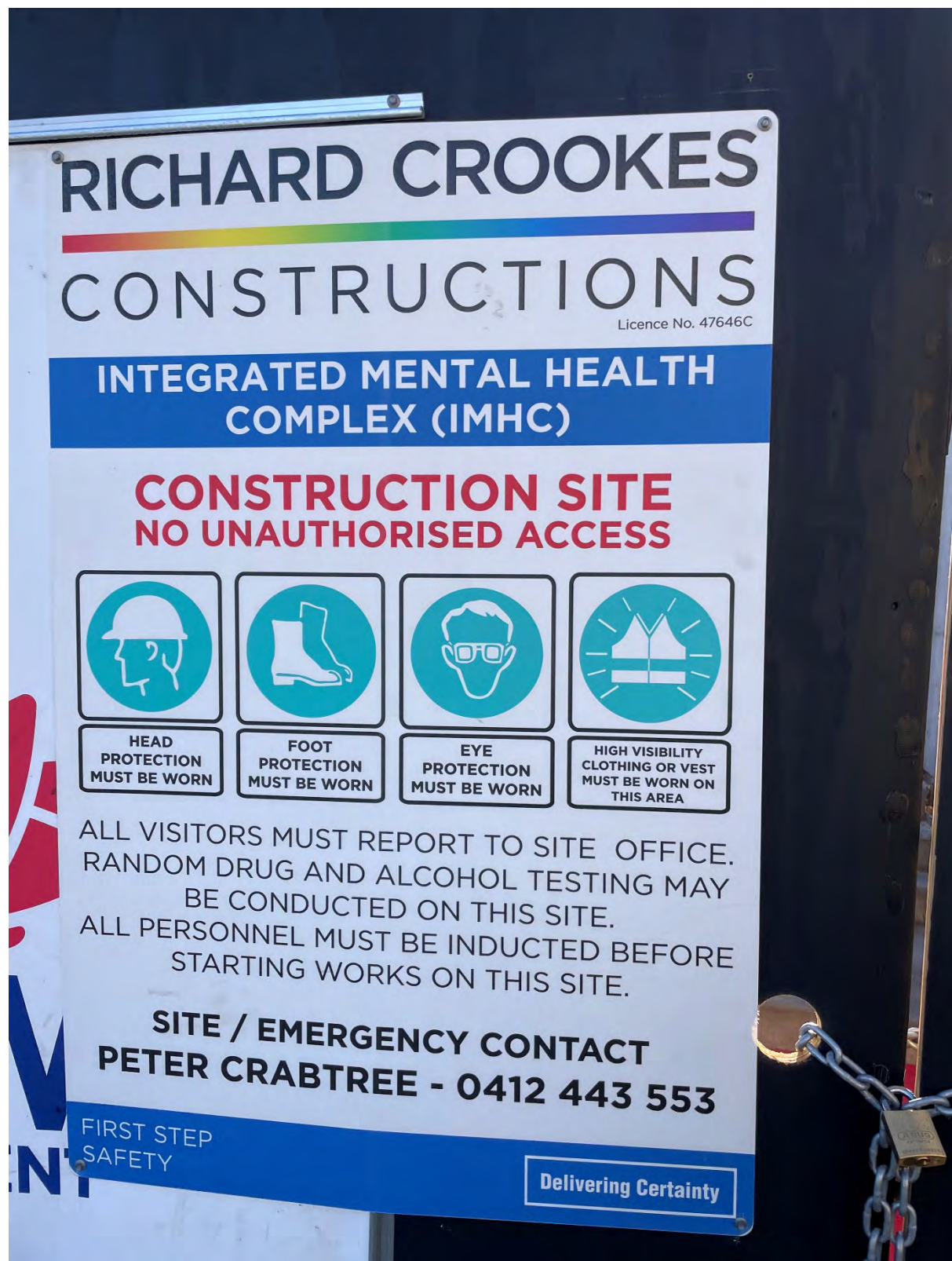
Figure 1 Project entrance site signage
