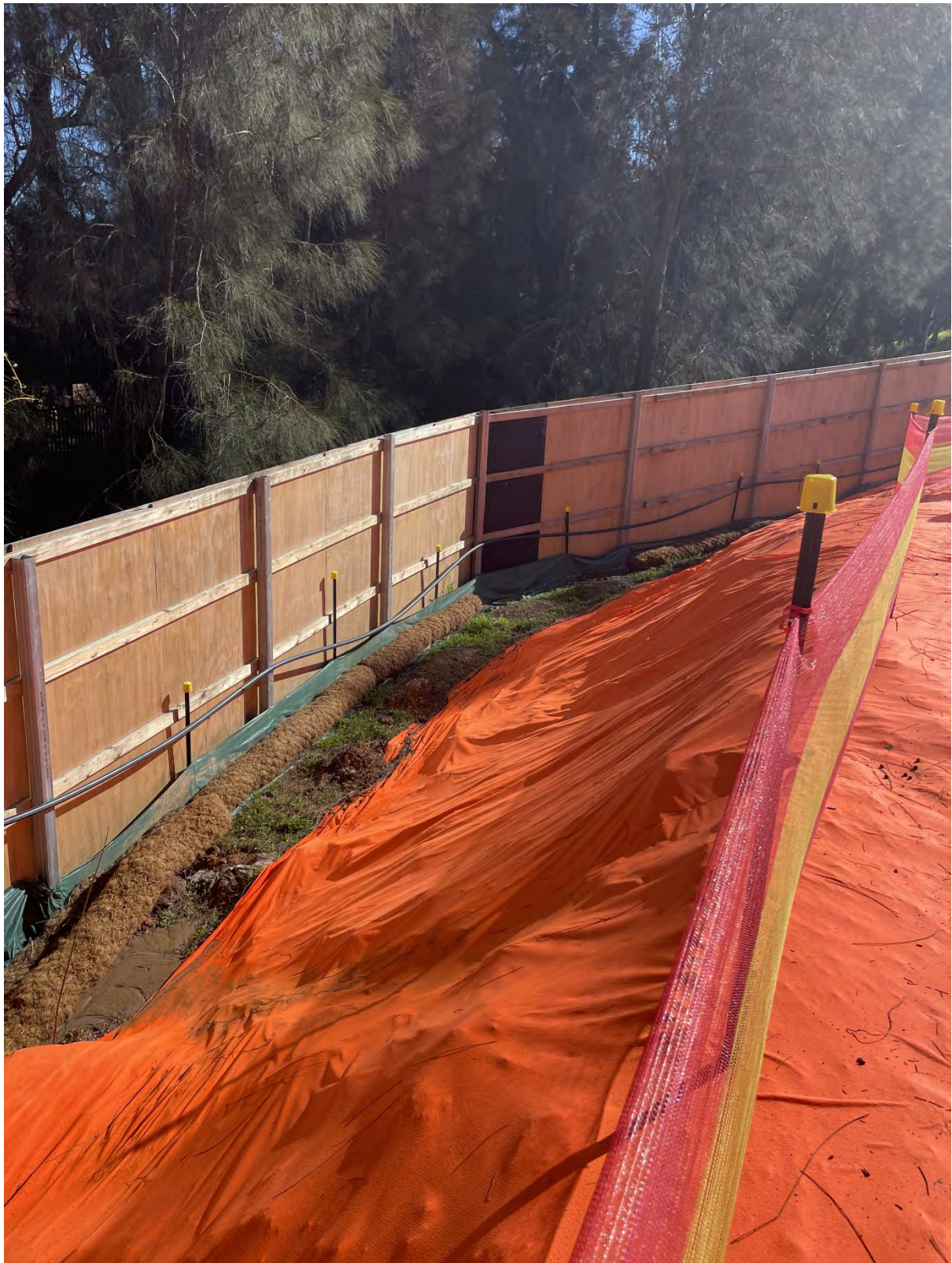
Figure 14 Sediment fence in place on site boundary
