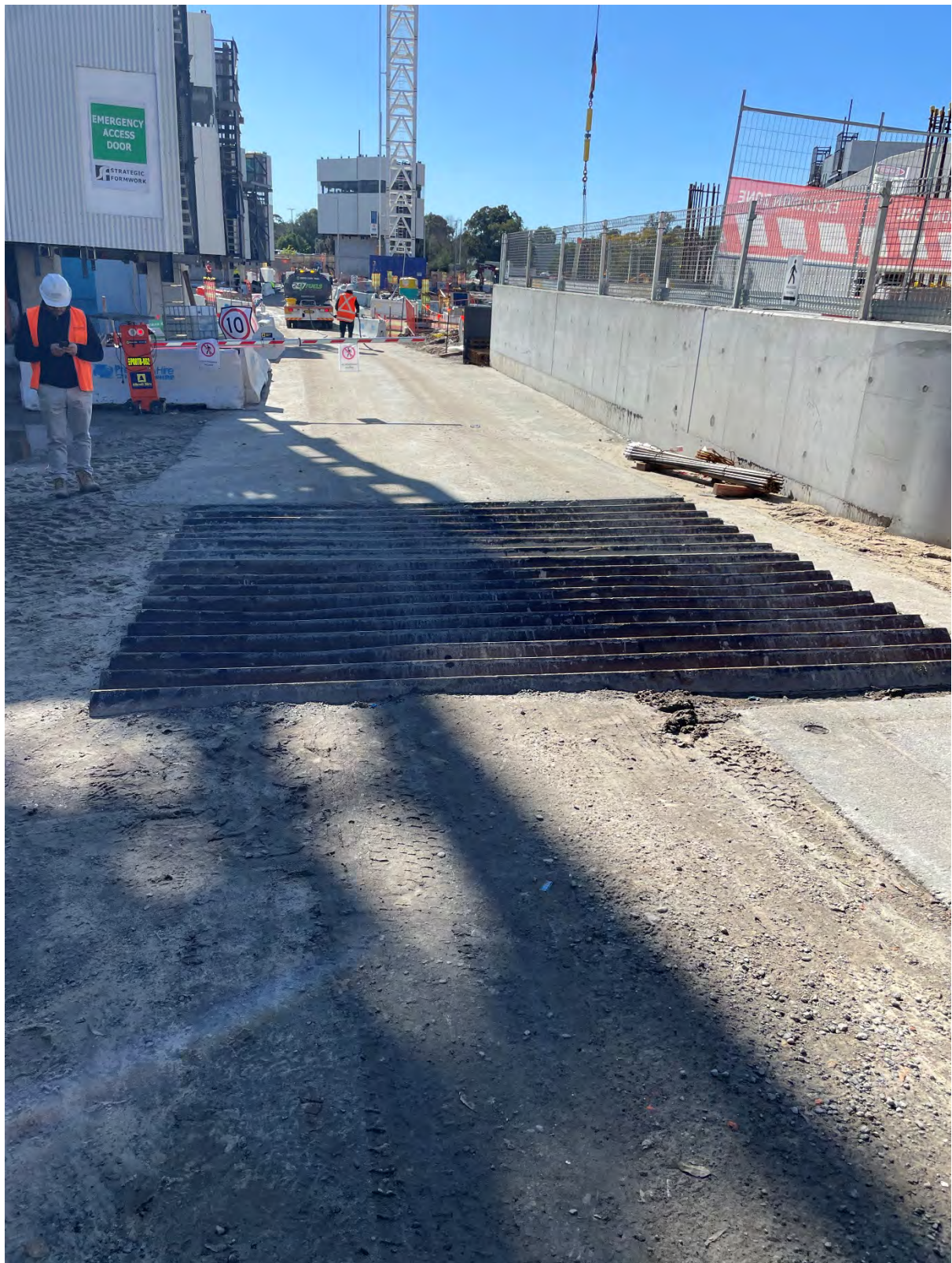
Figure 18 Site entry and exit with rumble grid and stabilised access
