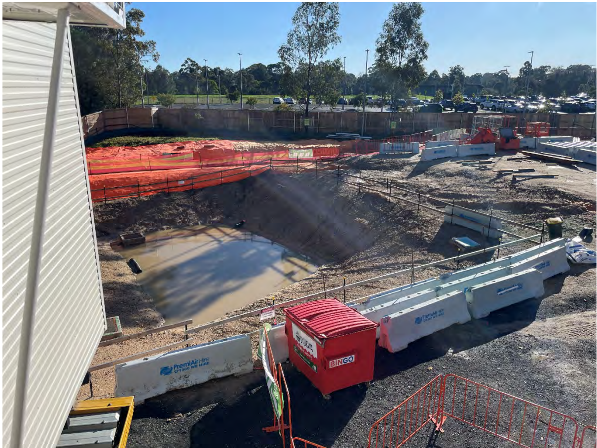
Figure 12 Onsite stormwater detention basin
