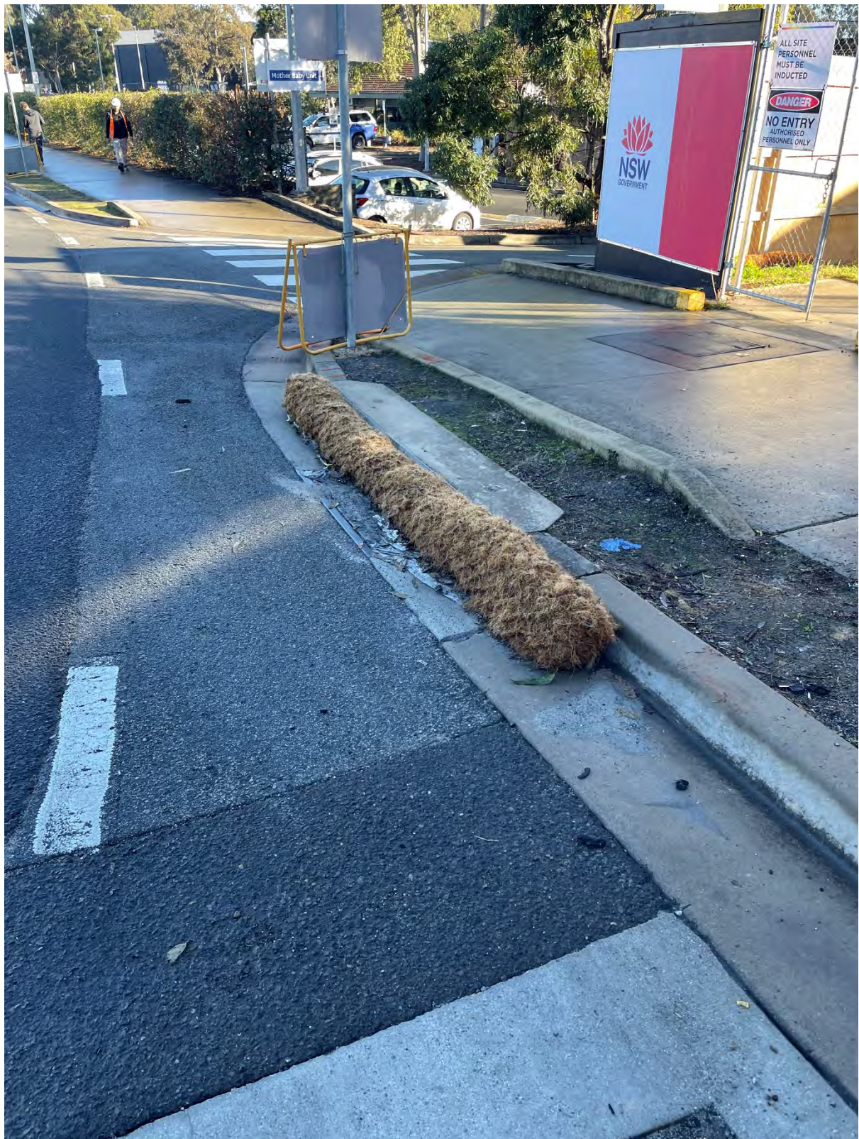
Figure 8 Sediment controls in place at stormwater drain
