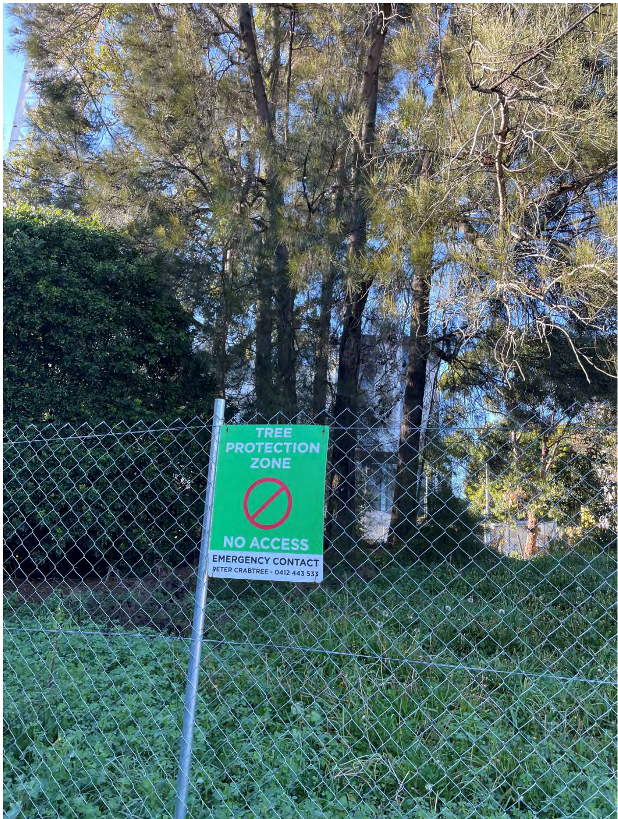
Figure 11 Tree protection zone in place
