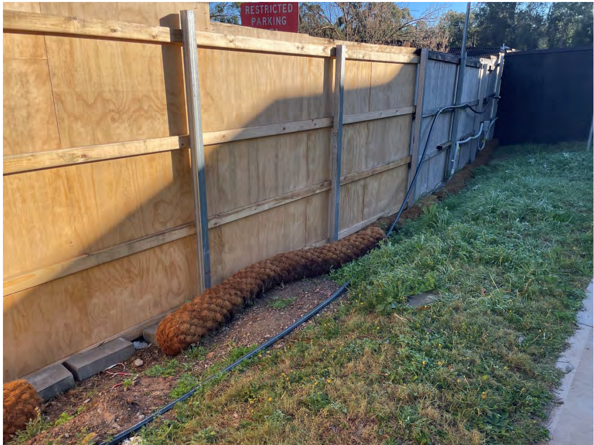
Figure 9 ERS&D controls in place on site boundary
