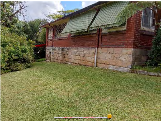
Photo 25 Facing northeast in 14 Bent Street showing residence disturbance
