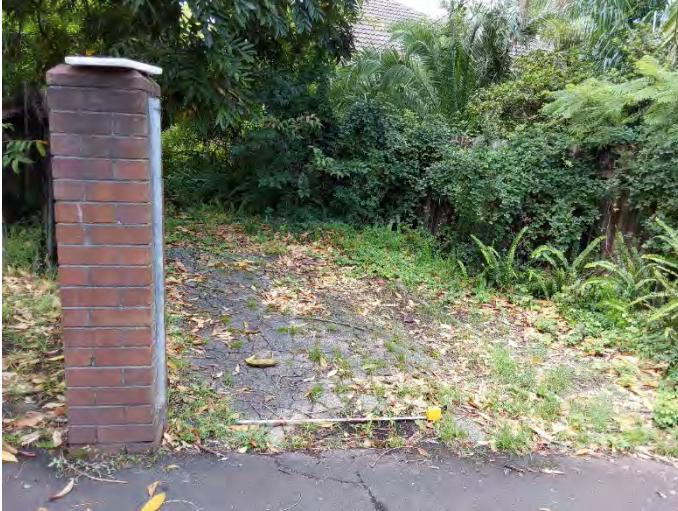
Photo 32 Facing south looking between 14 and 16 Bent Street showing driveway disturbance
