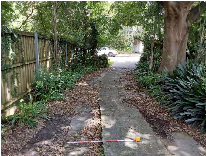
Photo 36 Facing north in 16 Bent Street showing driveway disturbance
