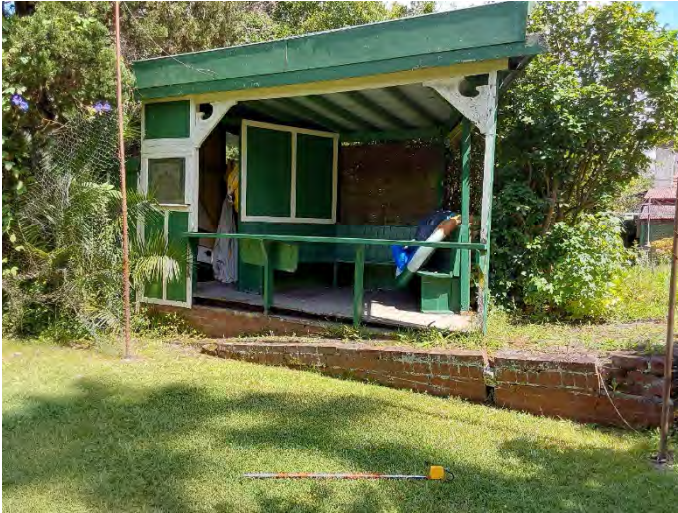
Photo 29 Facing northwest in 14 Bent Street showing disturbance from the construction of the tennis court
