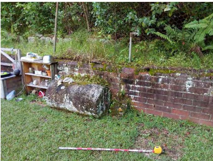
Photo 28 Facing northeast in 14 Bent Street showing disturbance from construction of the tennis court
