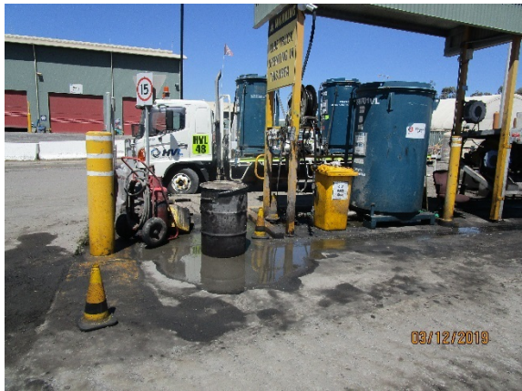
Photo 26. Hydrocarbon spill at the diesel re-fuelling area.
