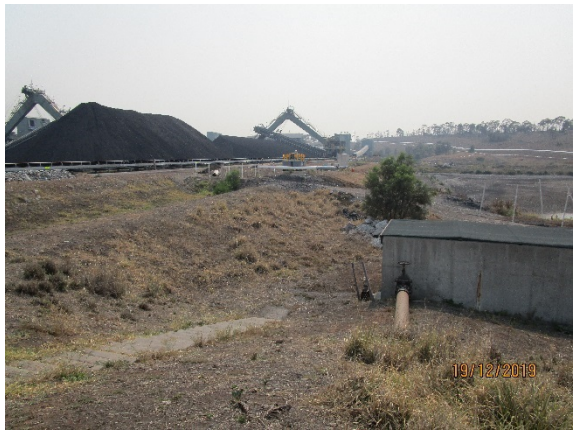
Photo 27. Coal stackers and waste water treatment plant (WWTP) dams.
