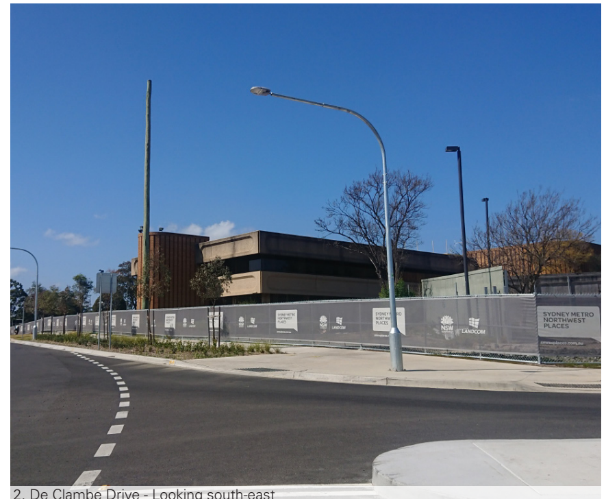
2. De Clambe Drive - Looking south-east
