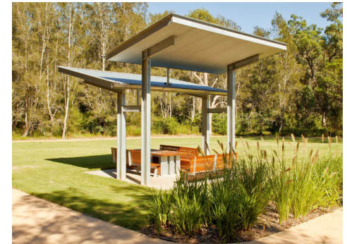
Figure 57: Picnic shelters and tables
