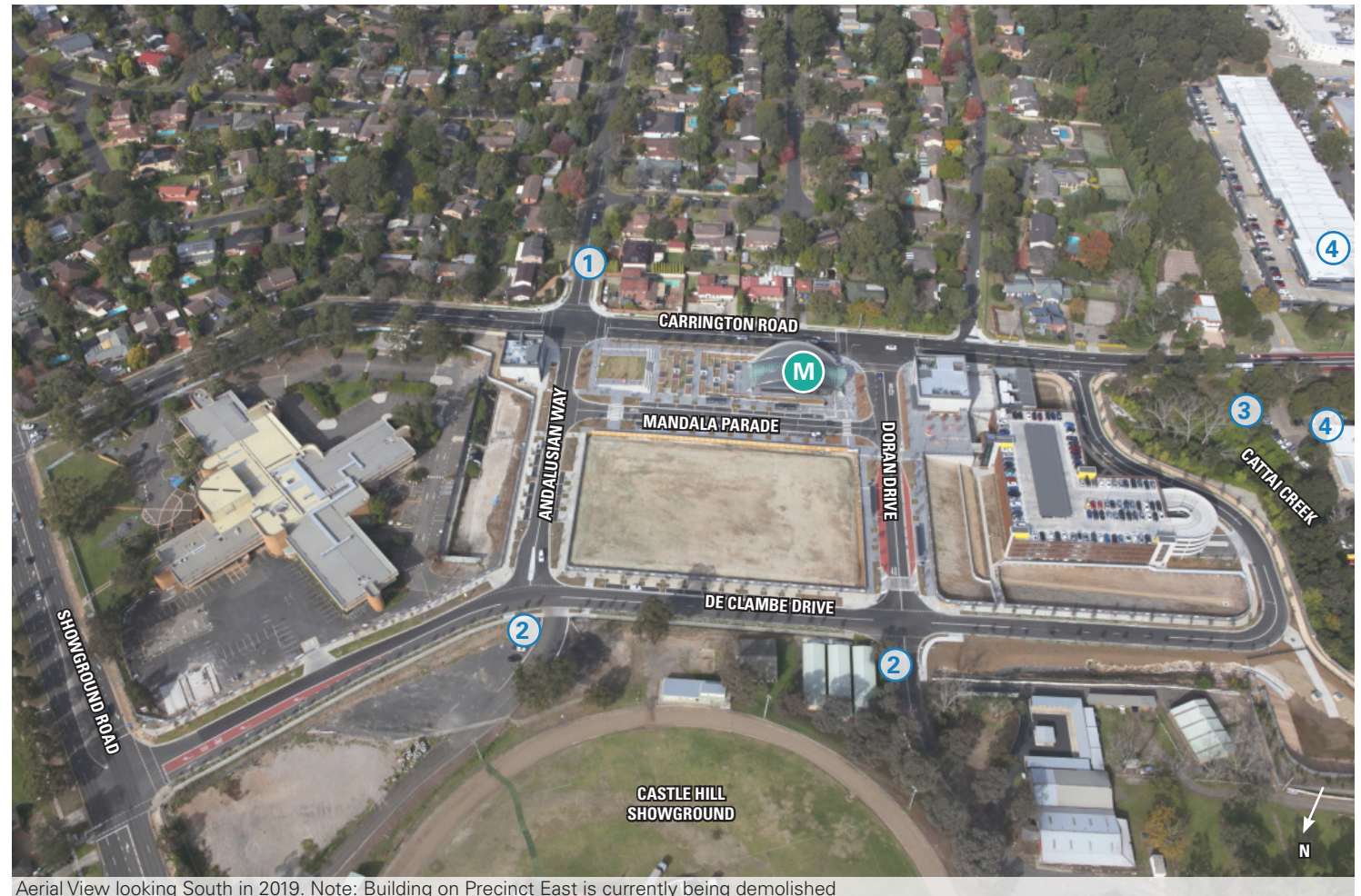
Aerial View looking South in 2019. Note: Building on Precinct East is currently being demolished
