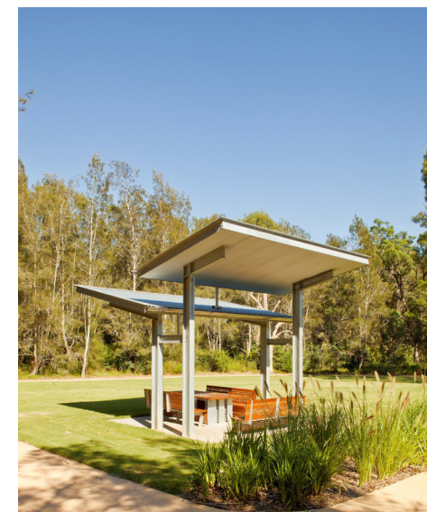
Figure 189: Picnic shelters and tables
