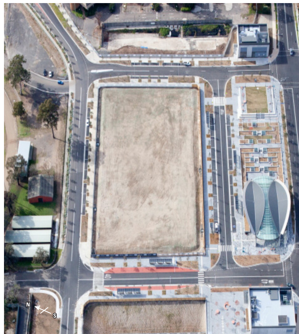
Figure 119: Doran Drive Precinct. Source: Sydney Metro 2019
