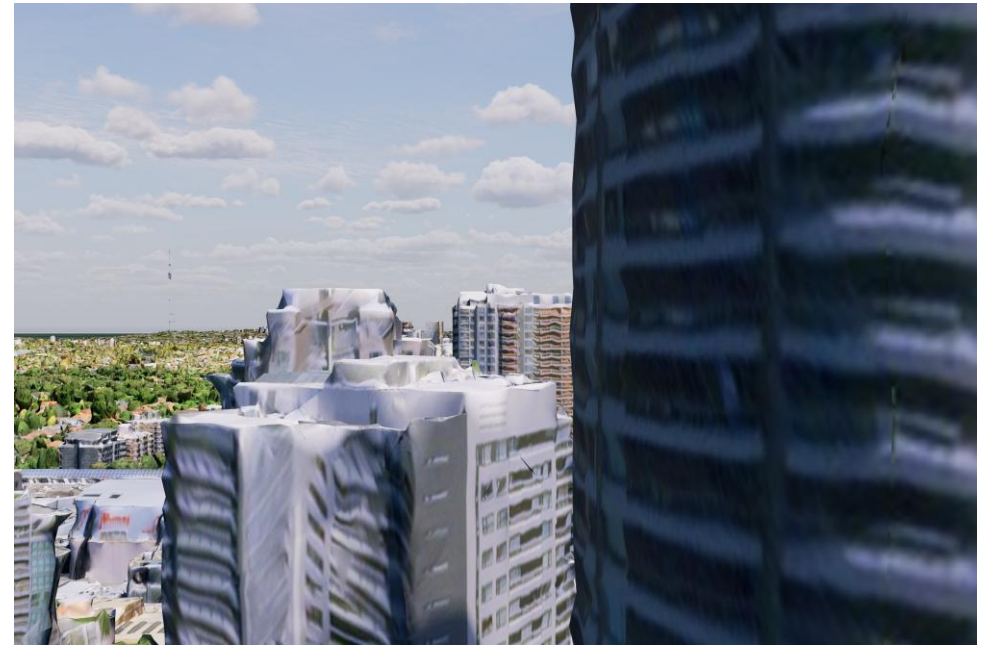
Figure 75 Altura, eastern elevation, upper levels (RL173), looking south, existing view
