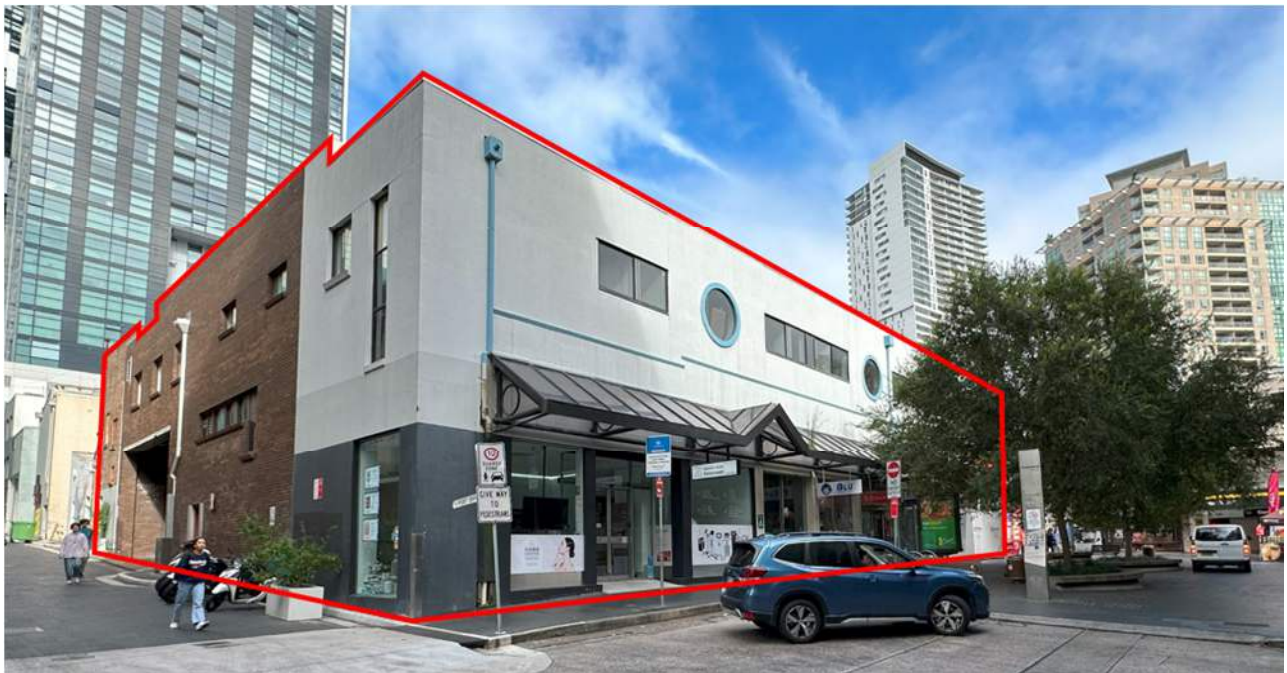
Figure 3 Existing Development to Victor Street Frontage (looking north-west, subject Site outlined red)
