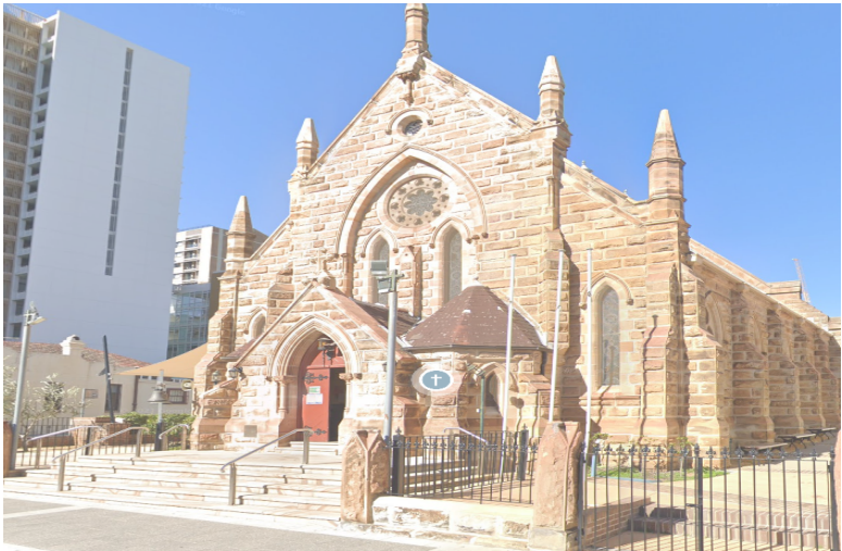
Adjacent heritage church
