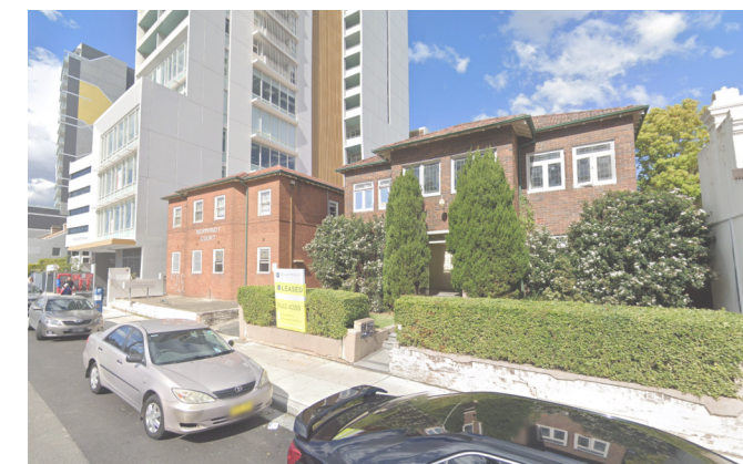
Residential flat buildings no. 18-18A Railway Pde
