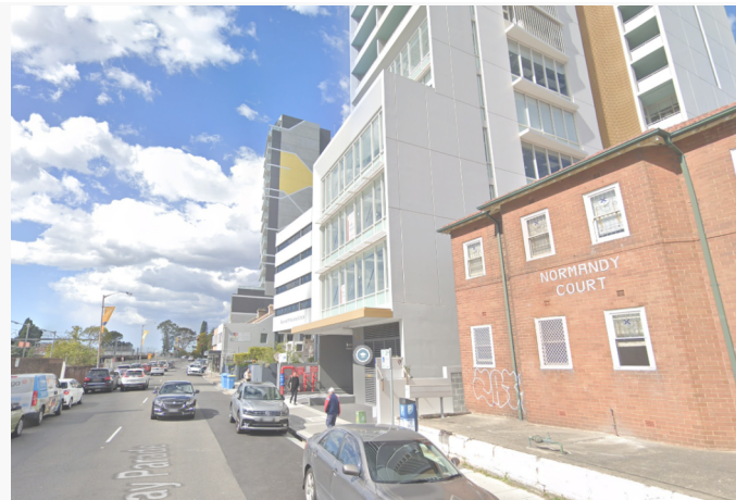
awning at 10-16 Railway Pde
