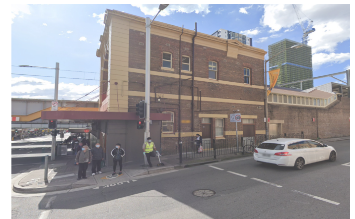
Item 2 - Burwood Train Station
