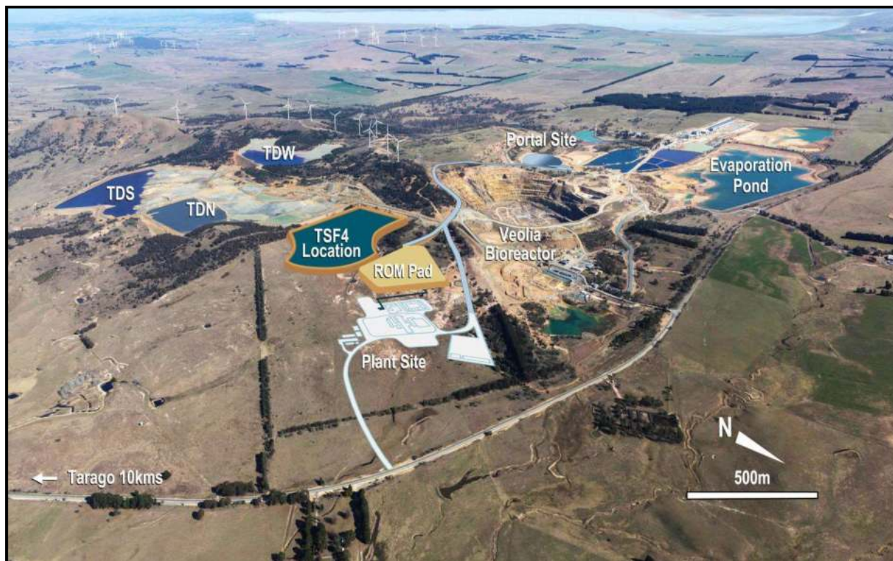
Figure 3.1 – Site Layout look to the south southwest
