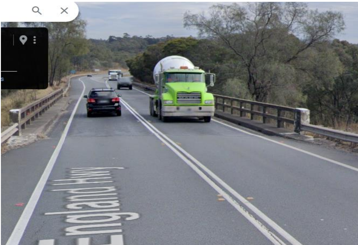
Narrow bridge approaching Power Station exit on New England Hwy
