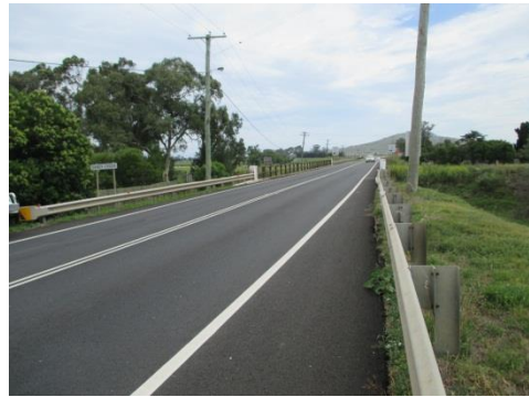
Sandy Creek Bridge, No obstruction
