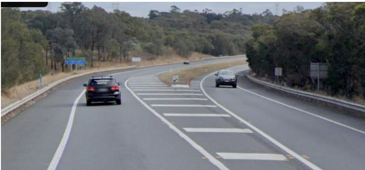
Start of divided road approaching Power Stations
