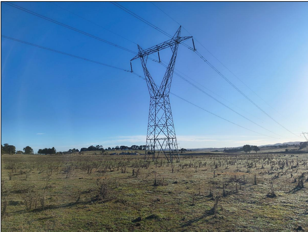
Plate 6: Built structures within the Project Area include an existing transmission line.
