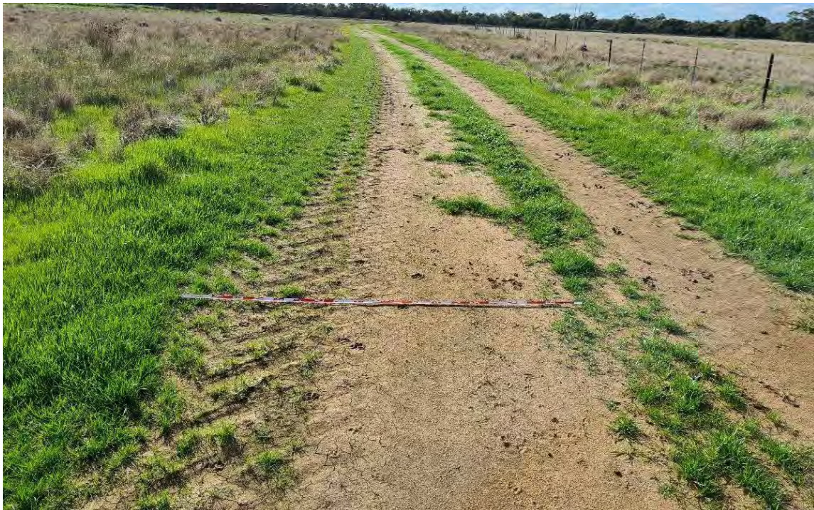
Figure 7.1 North-view of Hartwood Weir informal vehicle/proposed access track.
