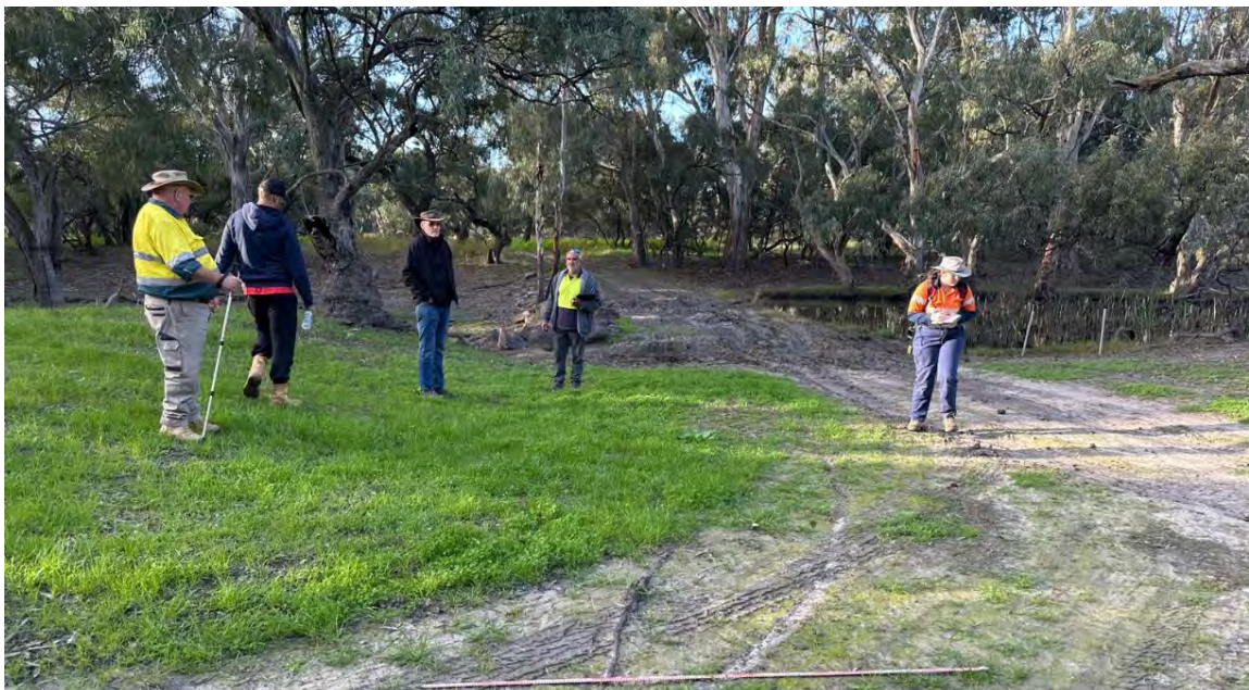
Figure 7.24 North-facing view of the proposed Forest Creek Block Bank construction zone.
