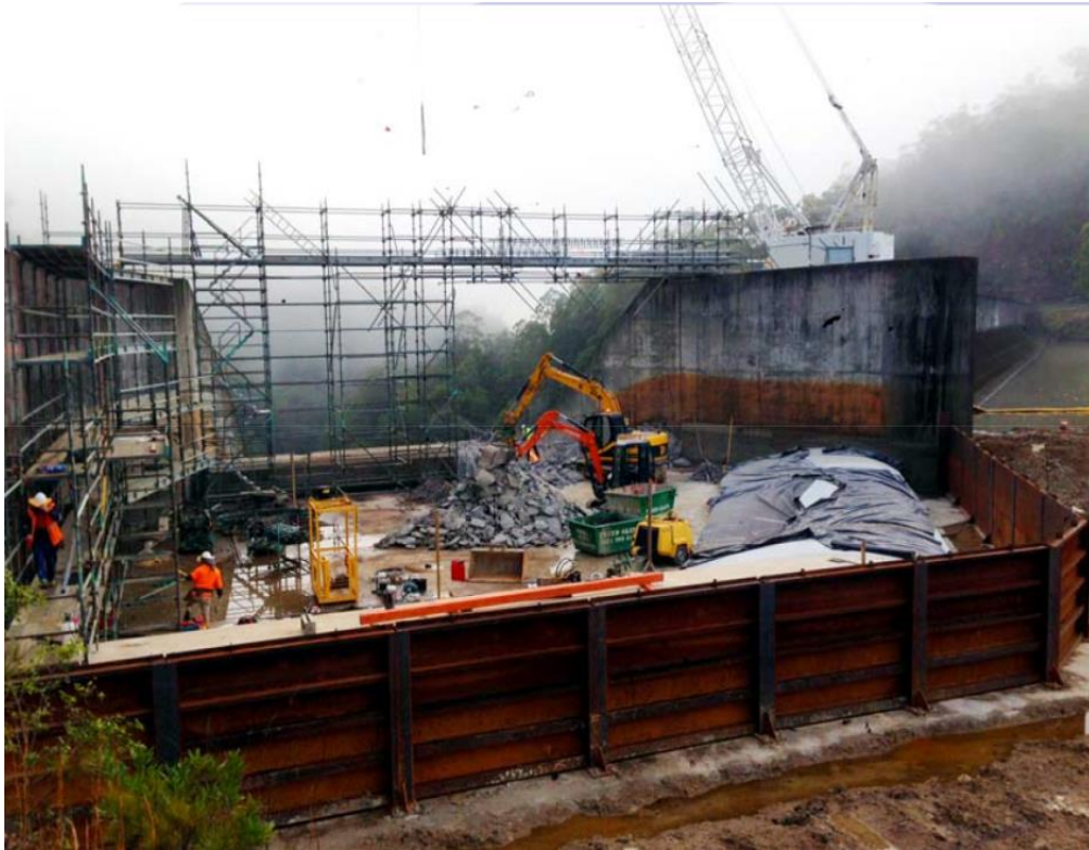
Photo showing construction of the spillway upgrade in 2013 (Source: Entracon bulletin Summer/Autumn 2013 Vol.2 Issue 4)
