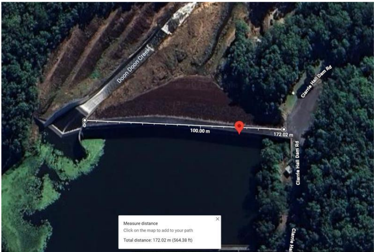
Figure 2-15: Existing Spillway and Dam (Source: Google Maps)
