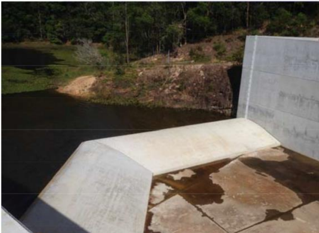
Photo showing the completed spillway crest (Source: Entracon bulletin Summer/Autumn 2013 Vol.2 Issue 4)
