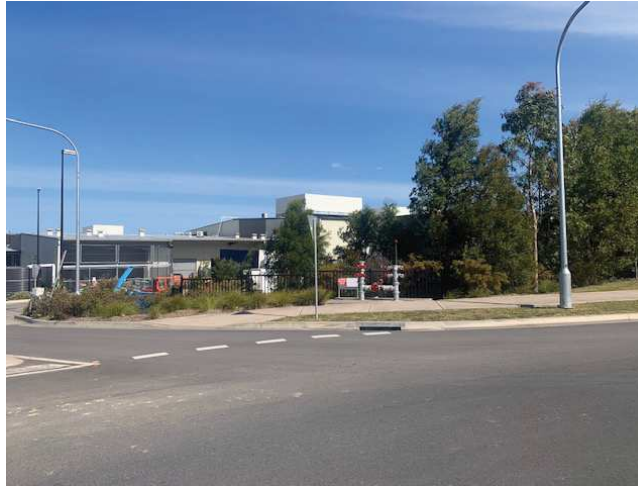
2. Photo looking SW across Moona Creek Road to the NE corner of the site. Sprinkler tanks are behind tallest trees visible in photo.
