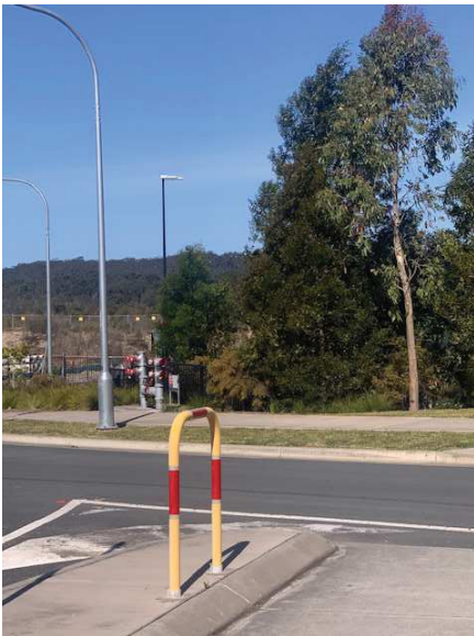
4. Photo looking SE with fire hydrant on the left and sprinkler tanks off the photo to the right.
