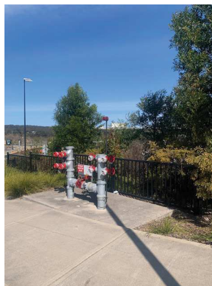
5. Close up photo compared to photo 5 (left). Close up of the fire hydrant. Also visible: existing fence.
