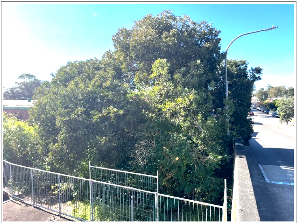
Figure 3 shows part of the stand required for removal to allow vehicular access.
